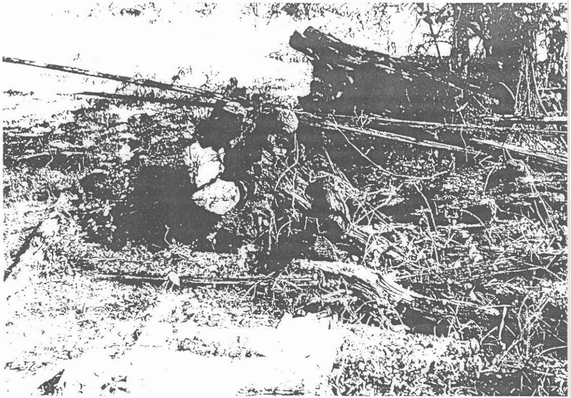
Figure 5A. The log crib structure northwest of the house was made of axe cut logs with saddle notches.
