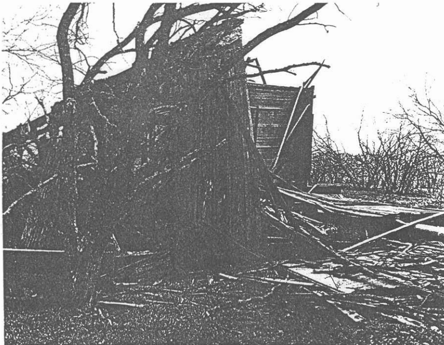
View of west end of house.
