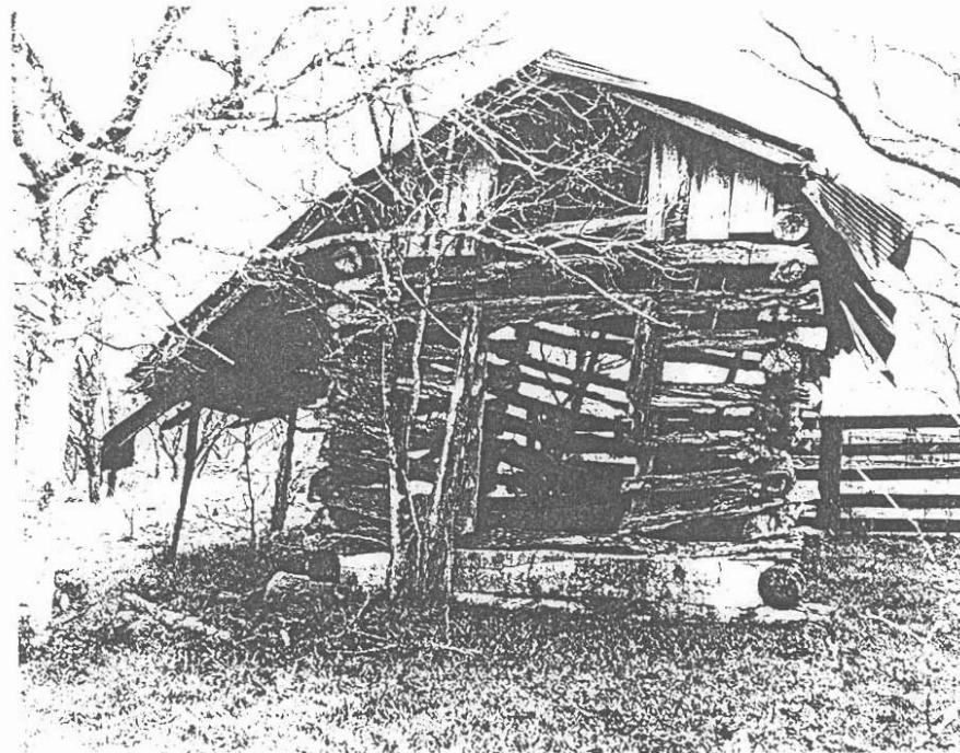
Front of log crib showing concrete "sill."
