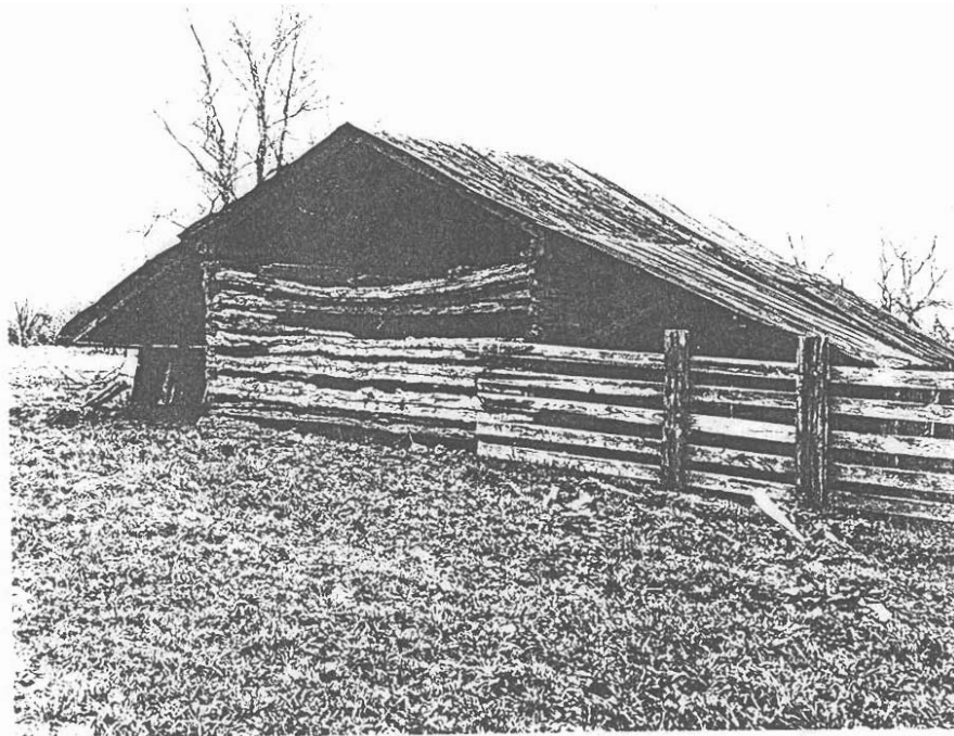
The south end of the large barn showing the original log construction and recent corrugated metal fence.
