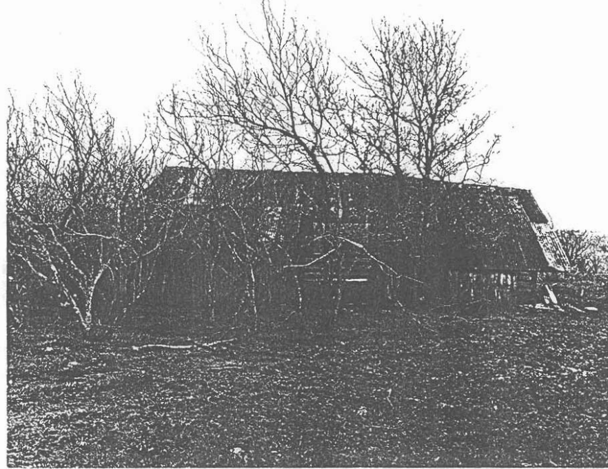
The large barn, located east of the house outside the SH 47 right-of-way. Looking east.
