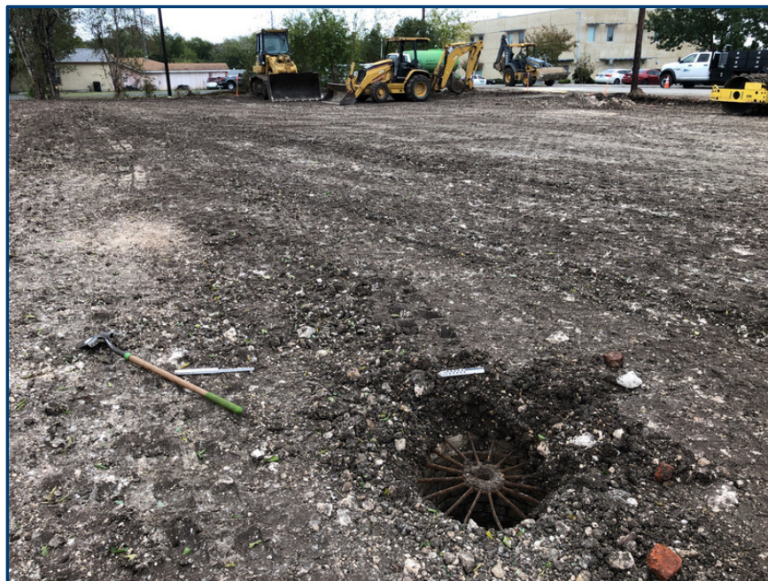
Figure 5. Overview of Parking Lot Location and Existing Construction Activities, Facing South.
