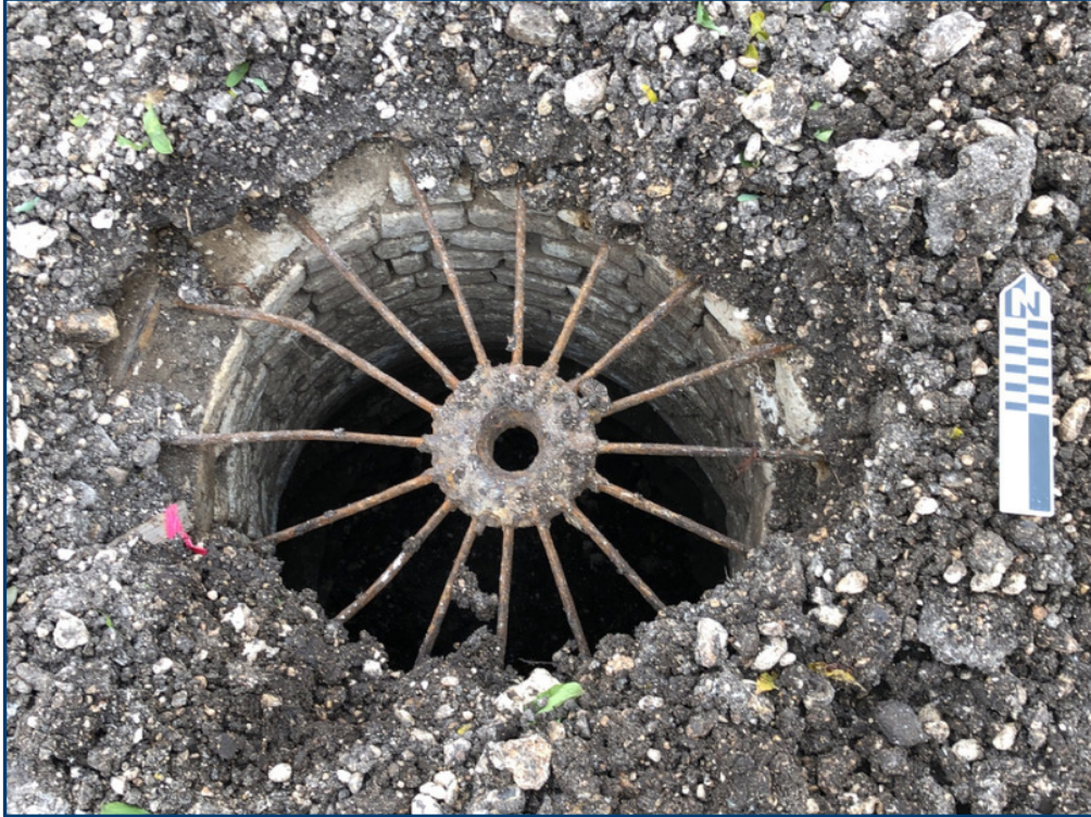
Figure 7. Cistern Opening, Facing North.
