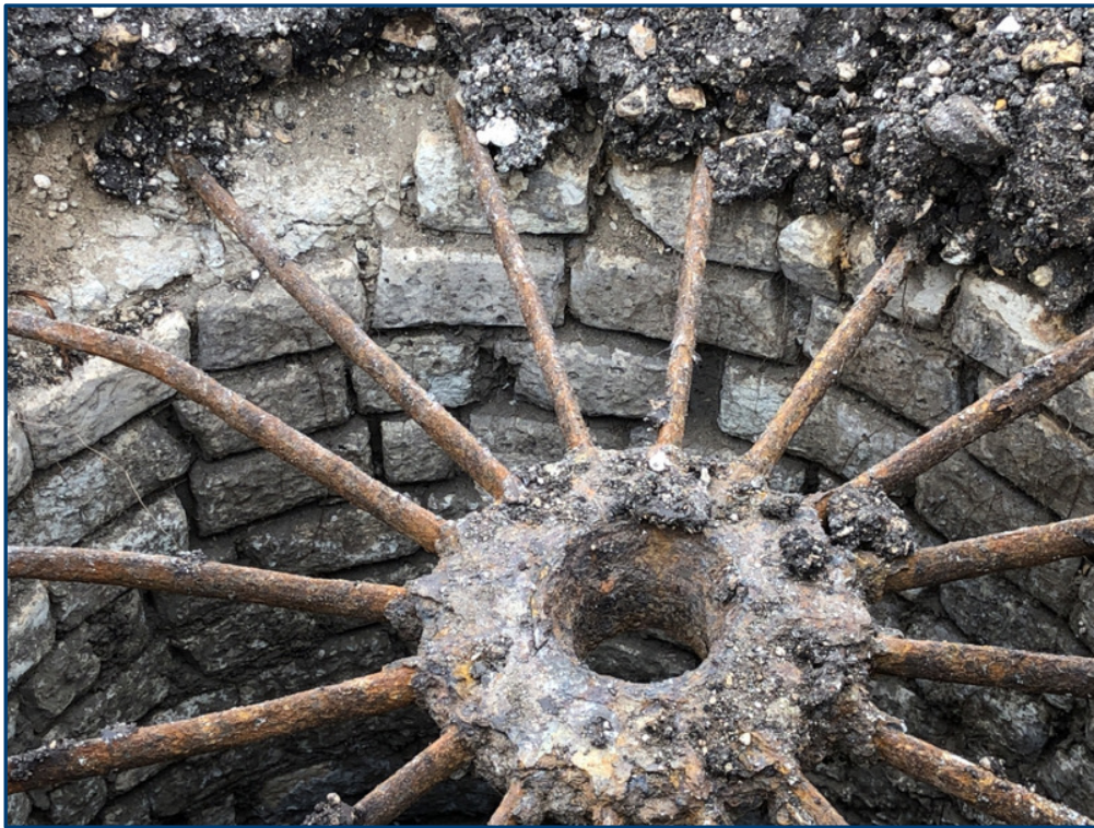
Figure 8. Cut Limestone Brick Lining Cistern, Facing North.
