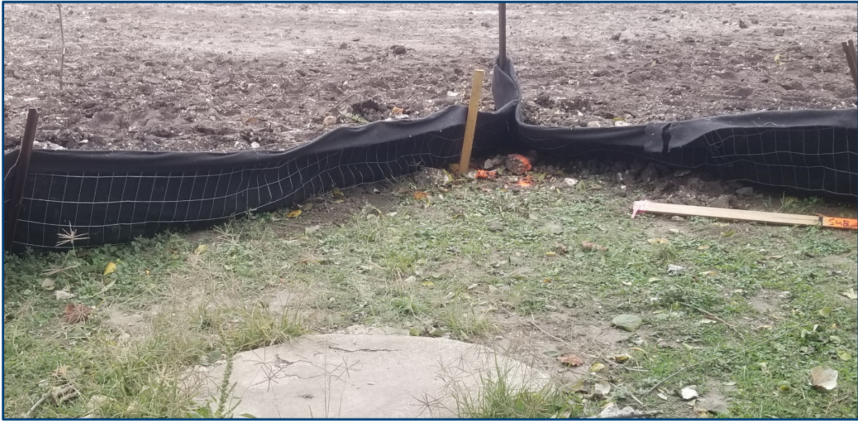
Figure 13. Overview of Single Grave Marker Location with Construction Fencing , Facing Southeast.
