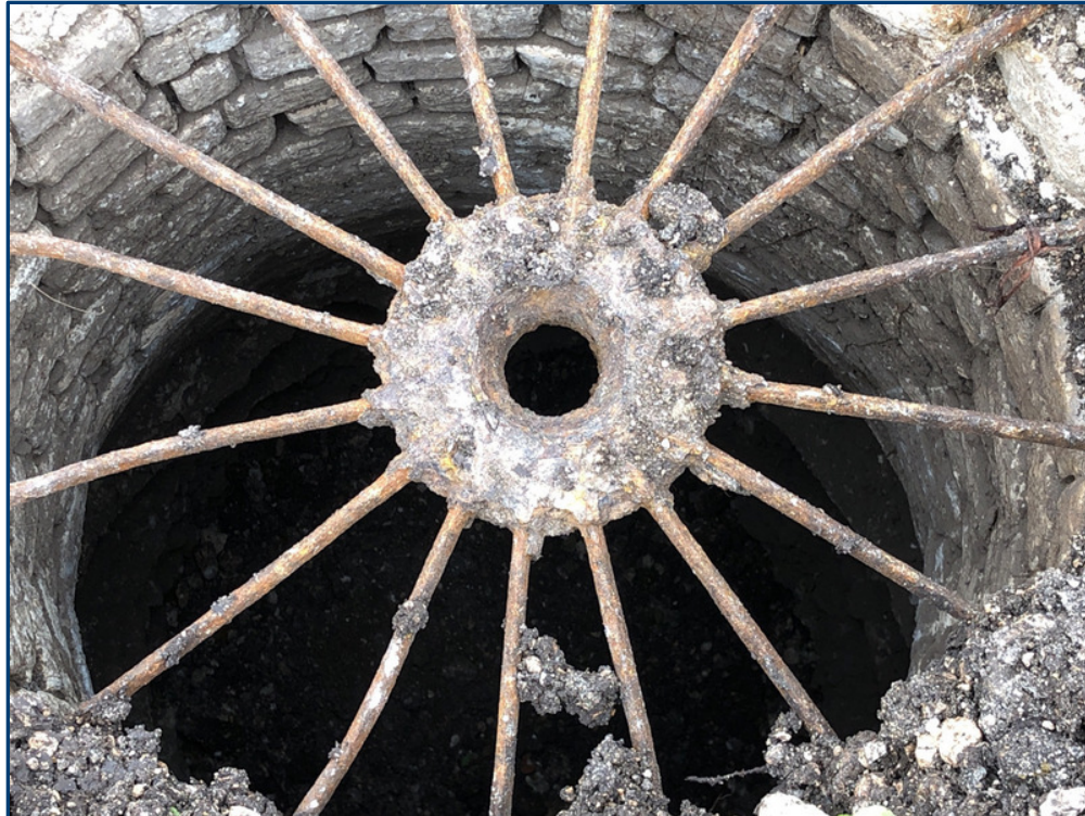
Figure 9. Cistern Interior with Accumulated Gravel at the Bottom, Facing North.
