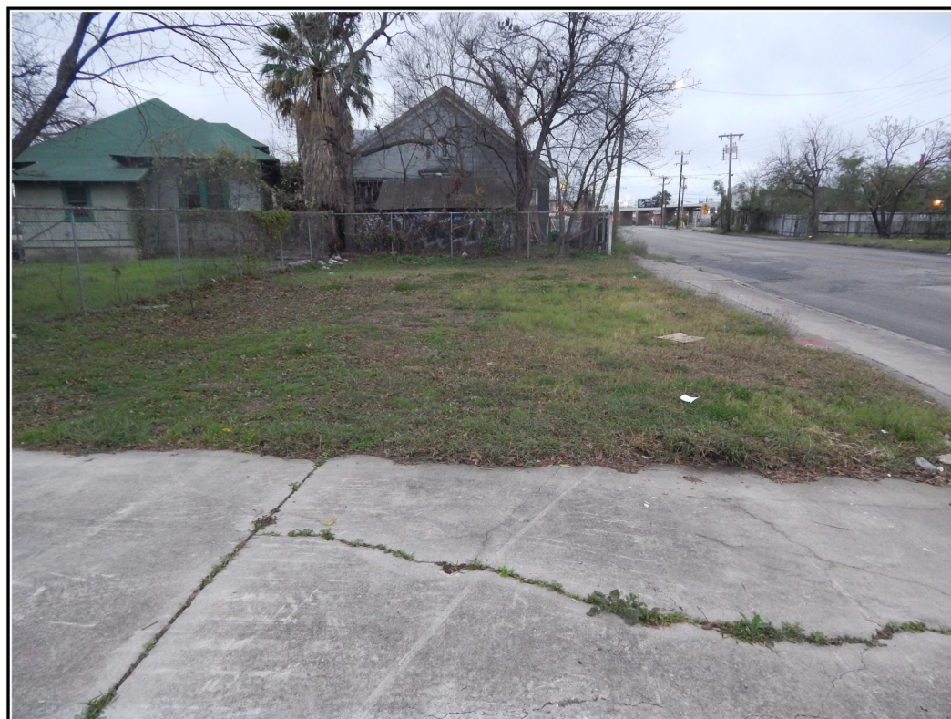
Figure 4-1. Project Area 1, prior to excavation. Facing east. Area is defined by the chain-link fence on the north and east, the sidewalk on the south, and the driveway (foreground) on the west.
