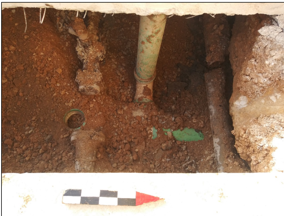
Figure 5-6. Construction gravels and utilities observed in the smaller trench, facing west.
