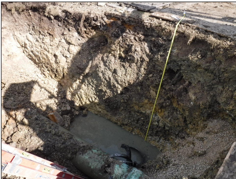
Figure 5-5. Maximum depth of BHT1, facing northeast.
