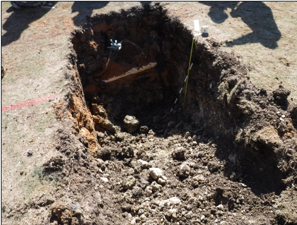
Figure 5-7. Previously installed utilities in BHT1, facing south.
