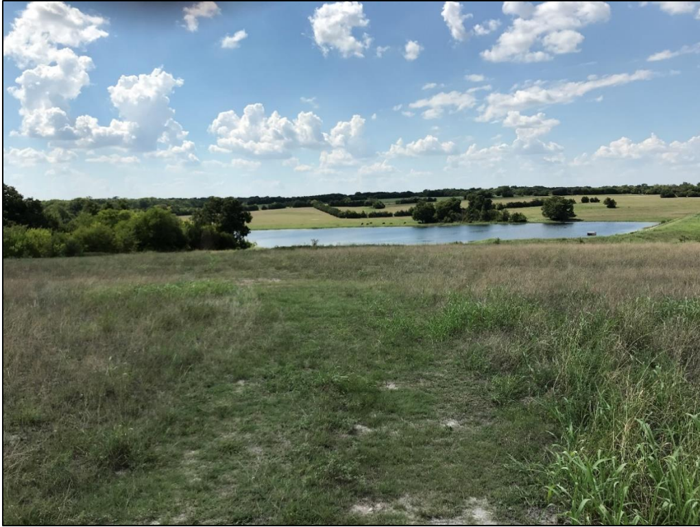
Figure 11. Transmission line easement east side of NRCS earthen dam (right) and SWCD Site 17 reservoir. Facing northwest.
