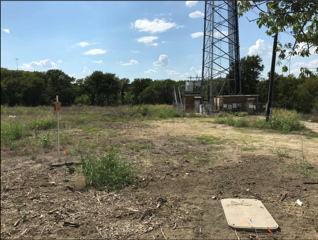
Figure 2. Transmission line easement west of Redbud Boulevard/CR 273 . Facing west.
