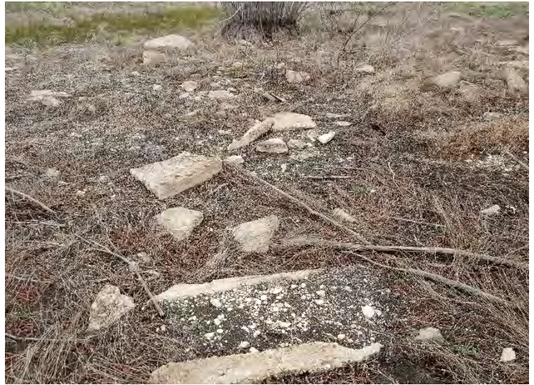
Photograph 14 – Inline PS APE, concrete debris in wetland, view to the north.
