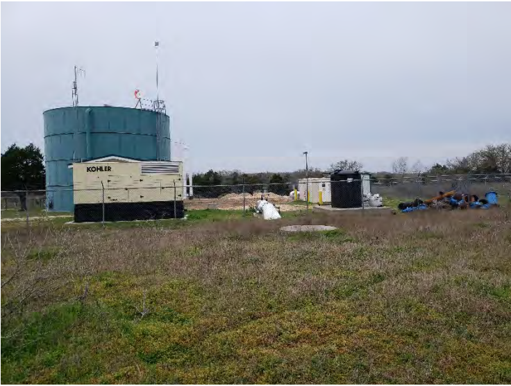
Photograph 25 – Shiloh PS facility, view to the northwest.
