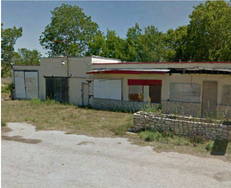
Photograph 1 – AR-1, 7361 FM 112, view to the north.
