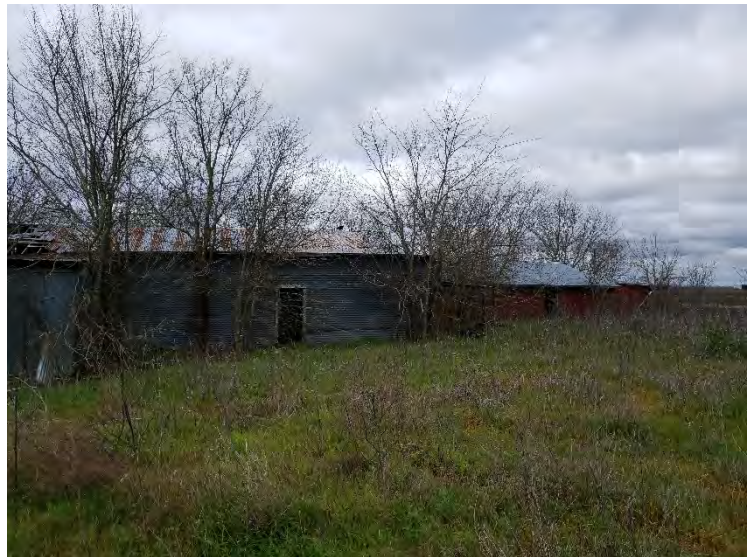
Photograph 10 – In-line PS APE, modern barn, view to the west.
