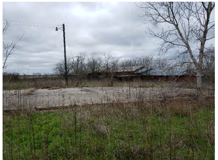
Photograph 30 – 41WM1419, Feature 1 historic-age building foundation, view to the southwest.
