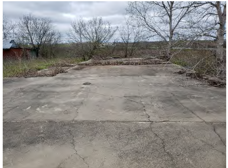
Photograph 36 – 41WM1419, Feature 1, view to the northwest.
