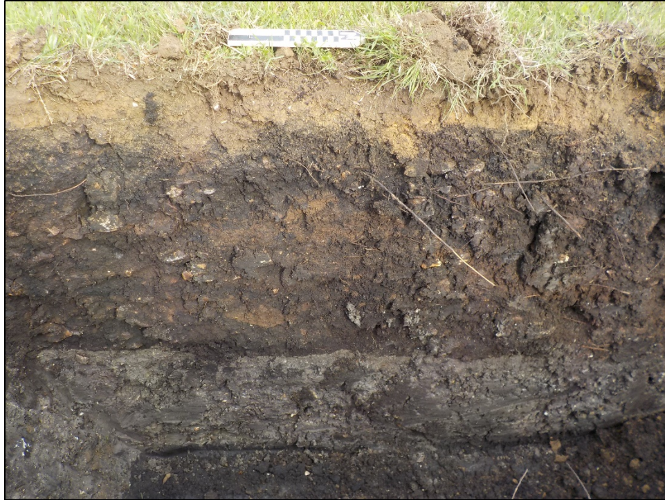
Figure 12. Overview of typical trench profile for Trenches 5–7 locale demonstrating disturbed soil over basal clay within the northern portion of the Project area, view facing west.
