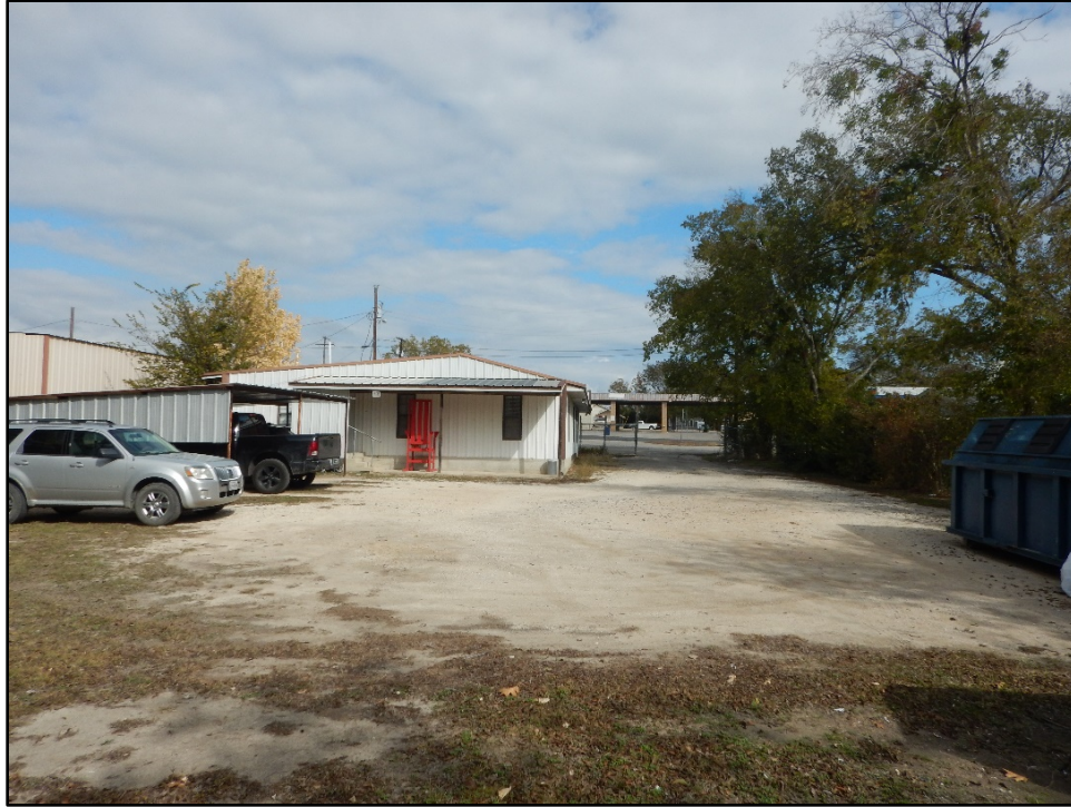
Figure 7. Example of extensive soil disturbance due to building, foundation, and parking lot construction.
