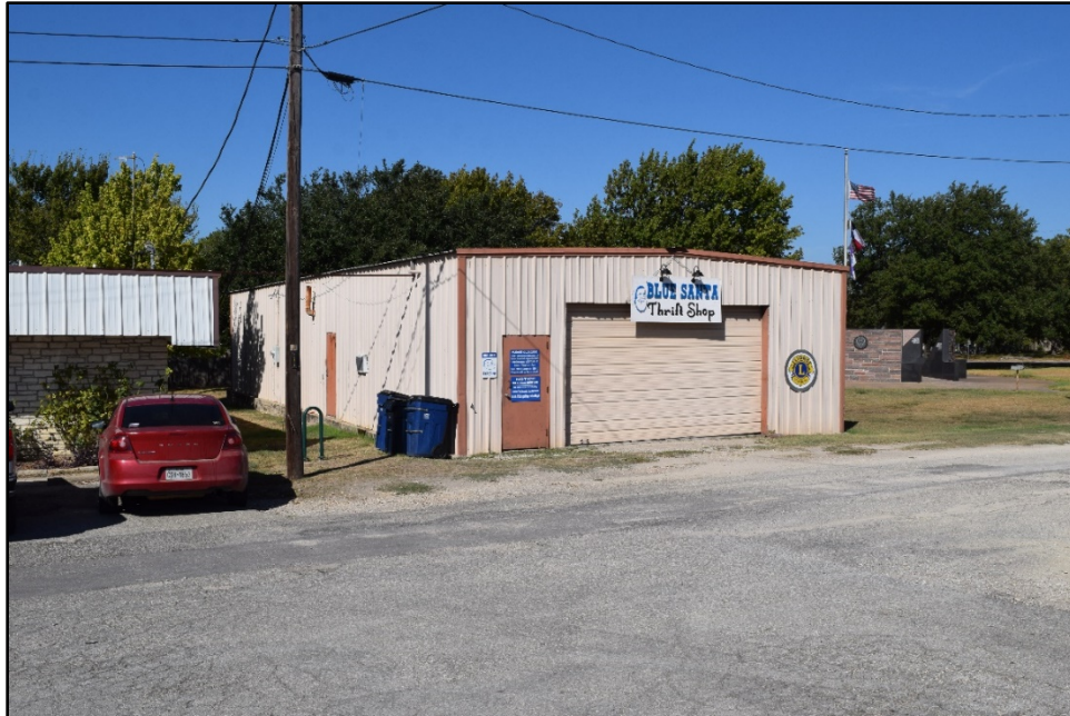
Figure 14. Storage building, oblique, east (front) and south elevations, facing northwest.
