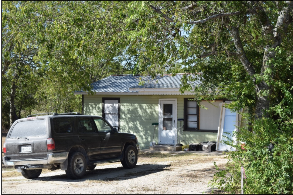
Figure 18. Historic-age residence immediately south of project area, east (front) elevation, facing southwest.
