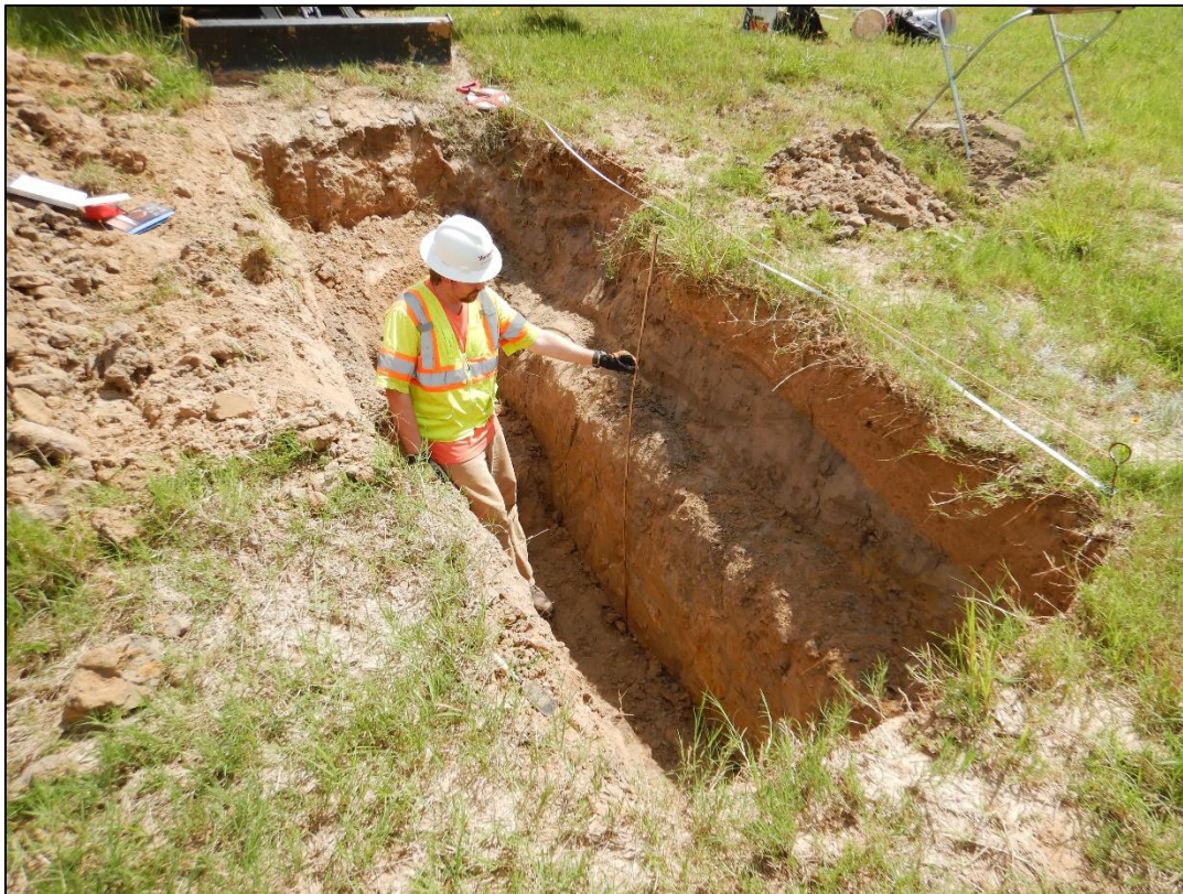
Figure 18. Trench 8 (facing northeast).
