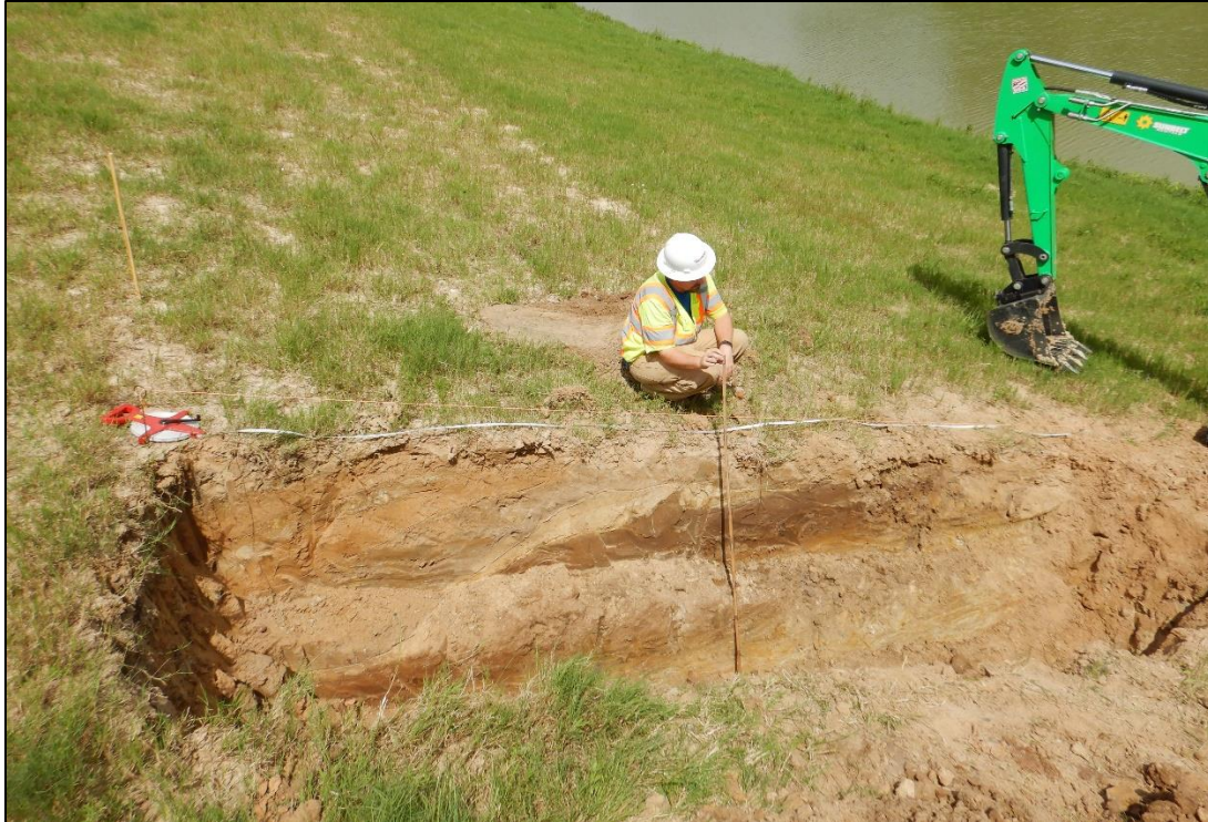
Figure 12. Trench 4 (facing west).
