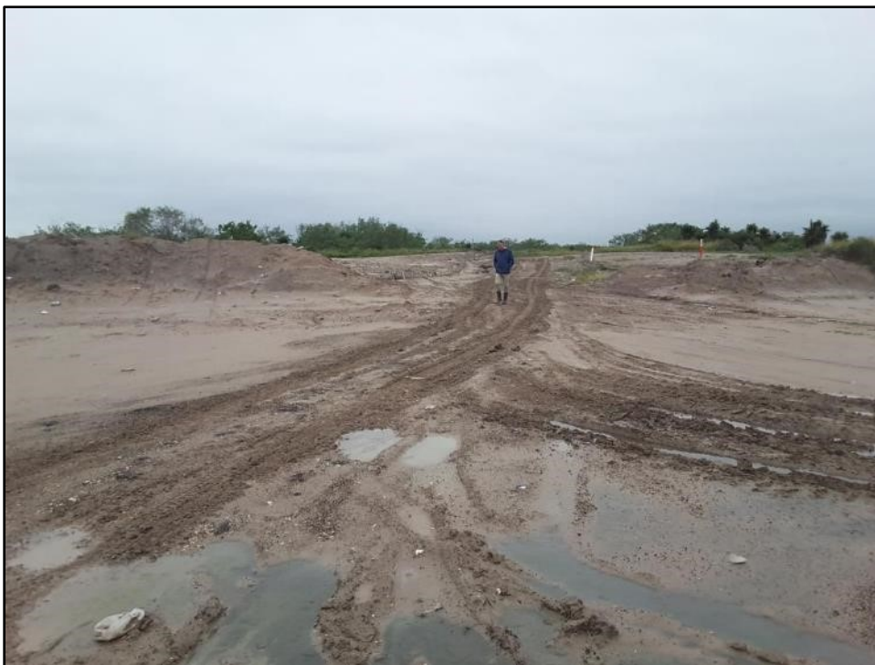
Figure 8. Existing access road on tract ND-CAM-082.000, facing south. Access road has long been in use for existing collocated pipeline marked by orange and white posts in background. Note wide road cut through low lomas near surveyor.
