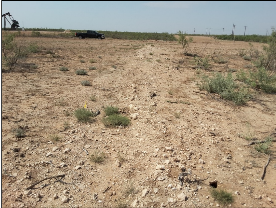
Figure 5. Overview of the southern terminus of Project area demonstrating completed construction, facing northwest.
