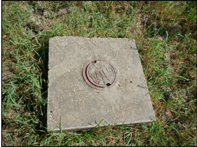
Figure 6.79. Close-up of modern manhole on 41GU176, facing east.
