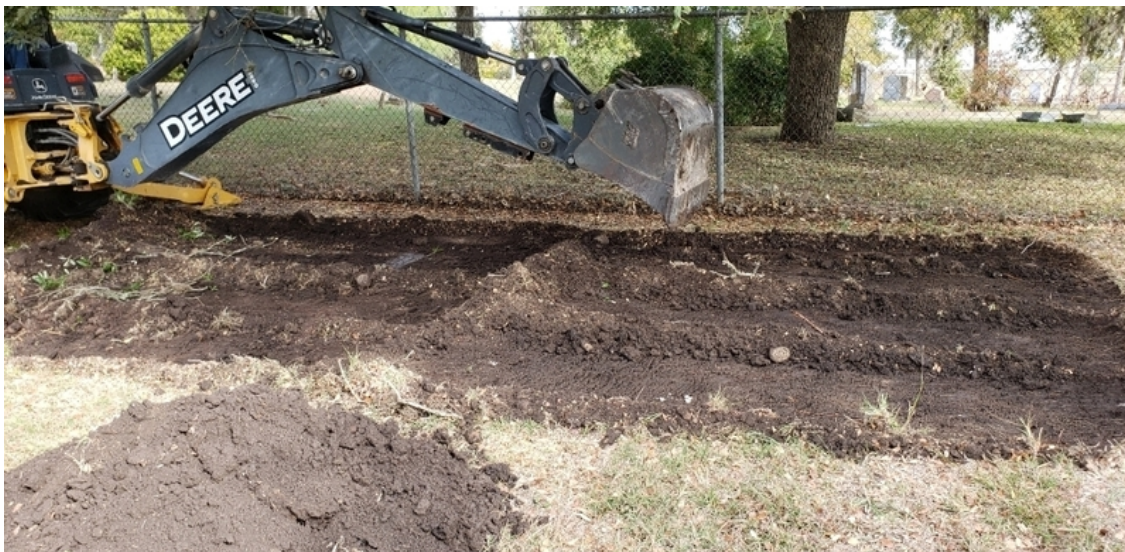
Figure 4-1: Overview of systematic mechanical scraping in progress, facing north.
