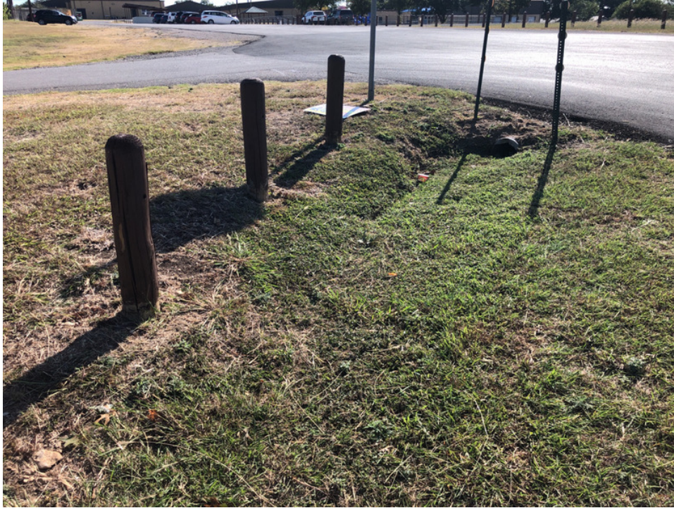
Figure 5-4: Overview of APE, facing east showing the survey end point and ground disturbance.
