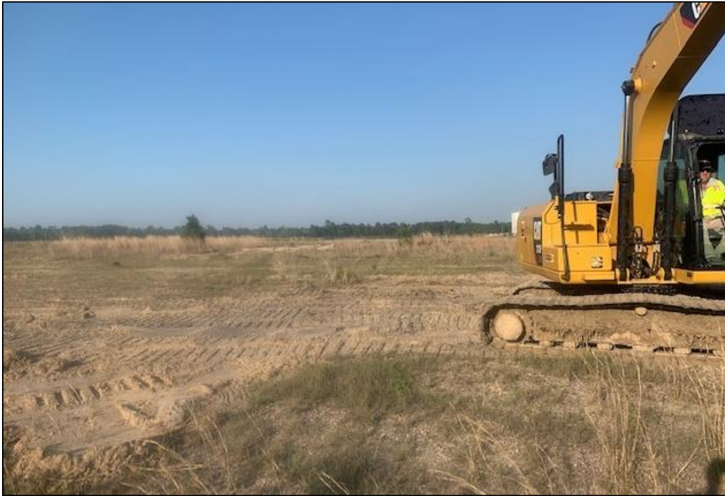
Figure A-20. Overview of Location of THT-7(Facing East)
