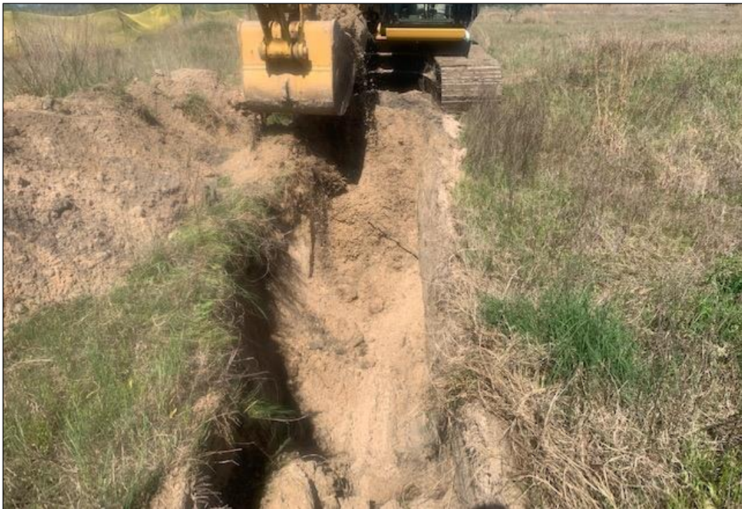
Figure A-9. Overview of THT-3 (Facing East)
