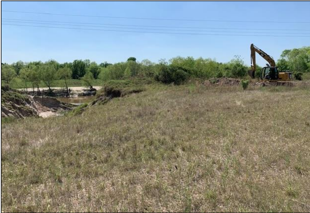
Figure A-5. Overview of Location of THT-2 (Facing West)
