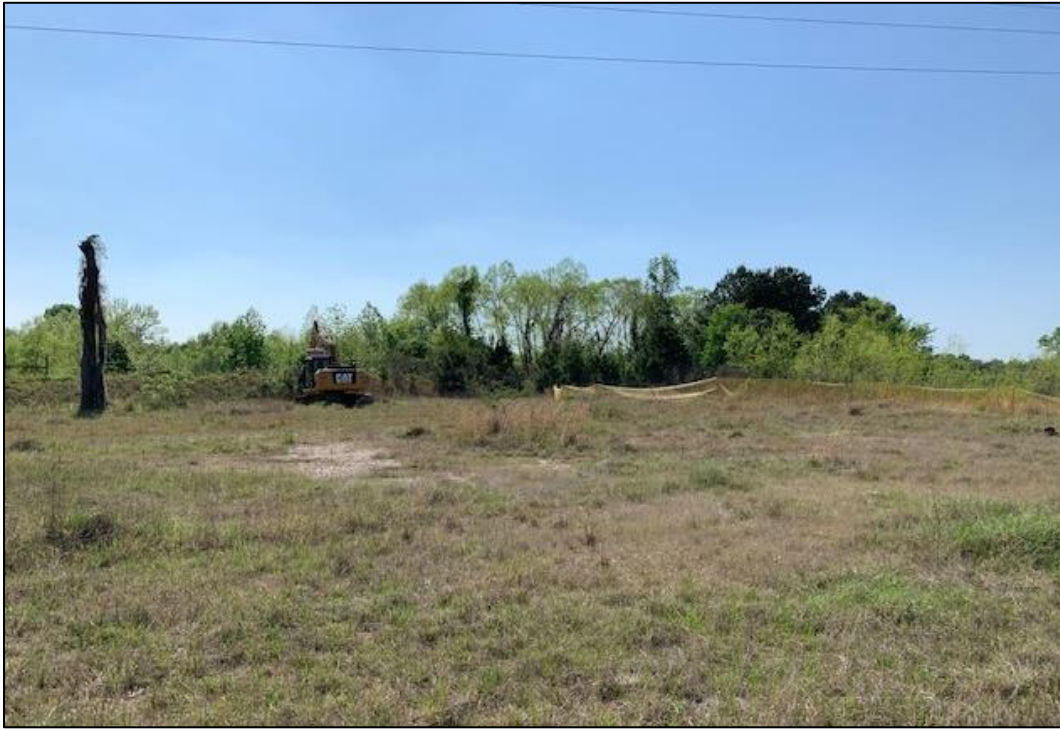
Figure A-8. Overview of Location of THT-3 (Facing East)
