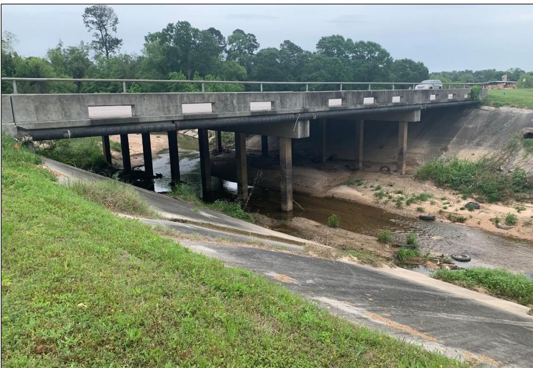
Figure 17. View of Stewarts Creek at Silverdale Drive Bridge (Facing Northeast)
