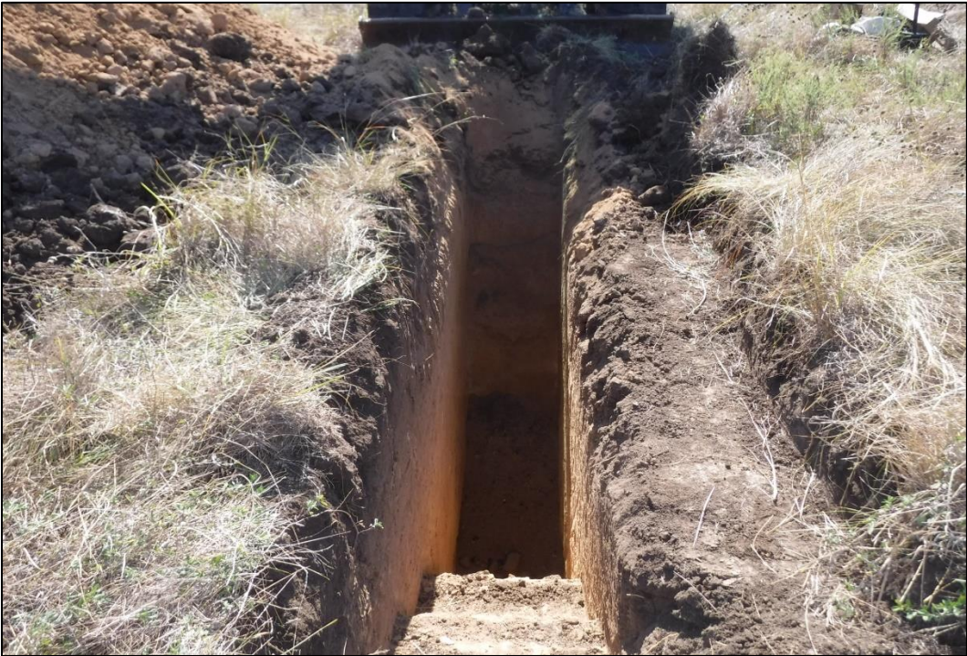
Figure B-3. Overview of BHT-2 (Facing South)
