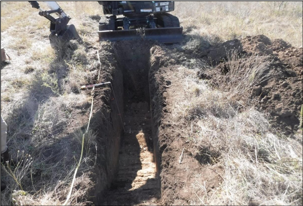
Figure B-1. Overview of BHT-1 (Facing South)
