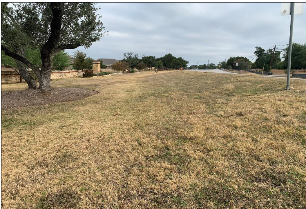
Figure 19. Eastern Portion of Reclaimed Water Line Paralleling FM 12 (Facing North)
