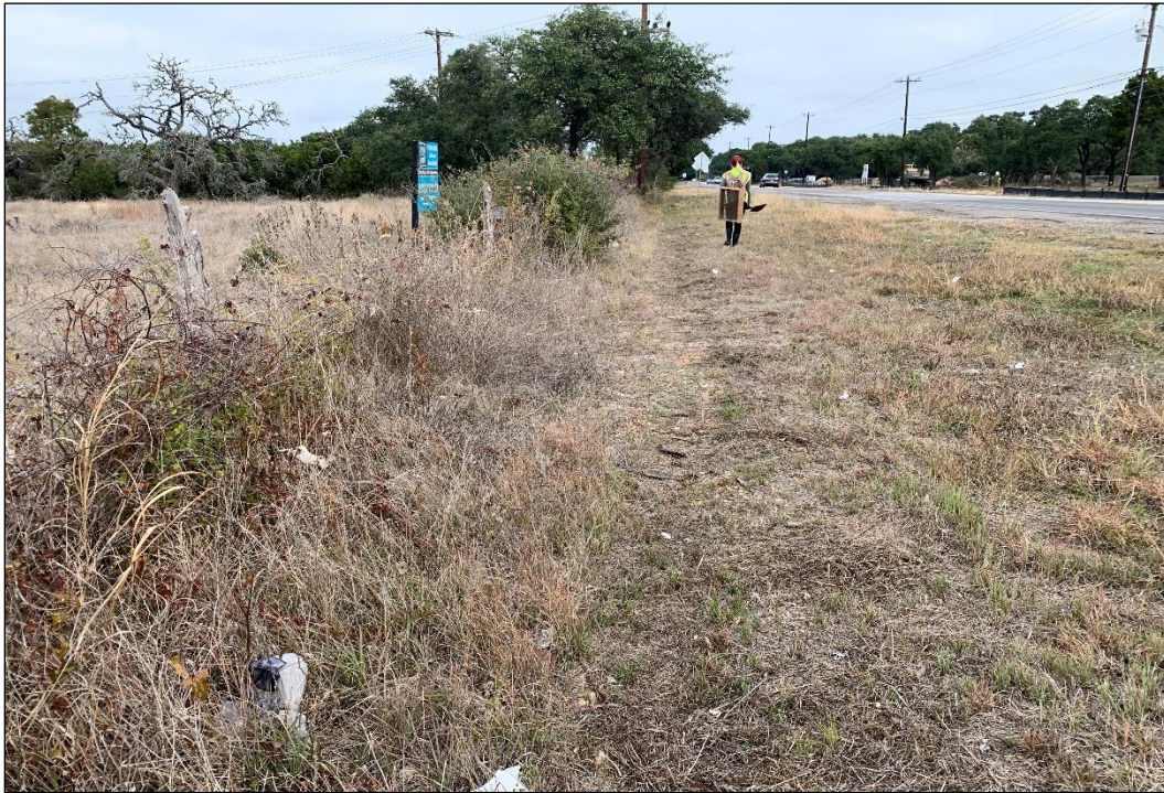
Figure 18. Eastern Portion of Reclaimed Water Line Paralleling FM 12 (Facing North)
