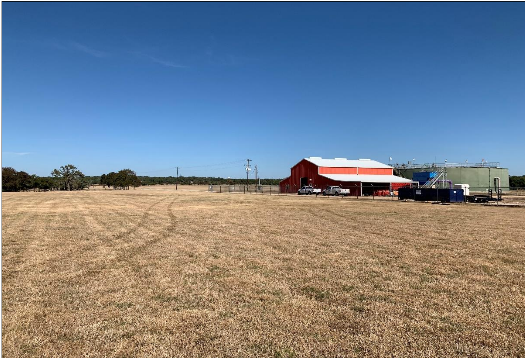
Figure 21. Existing Water Reclamation Facility Expansion Area (Note Existing Reclamation Facility at Right) (Facing North-Northeast)
