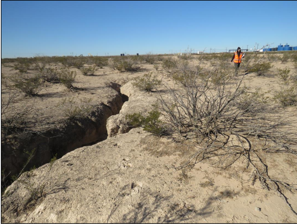
Figure 35: Erosional cuts common at site 41RV209, looking east.
