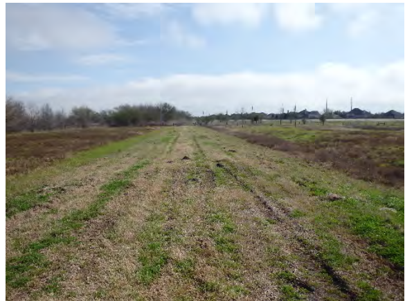
Figure 5-4. Levee road with inundated ditches at the western end of the APE. View is to the northwest.
