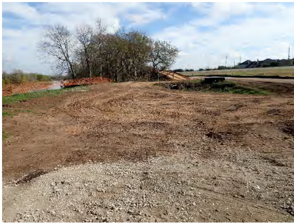
Figure 5-6. Workspace 3 with pre-existing culvert and drainage. View is to the east.
