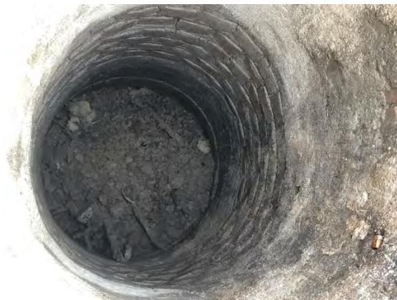
Figure 9-3. A view of the interior of Feature 6.
