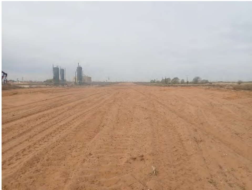
Figure 5-9. Overview of active pipeline work taking place within the southern half of Site 41MD58 at the time of delineation survey. View is to the east.
