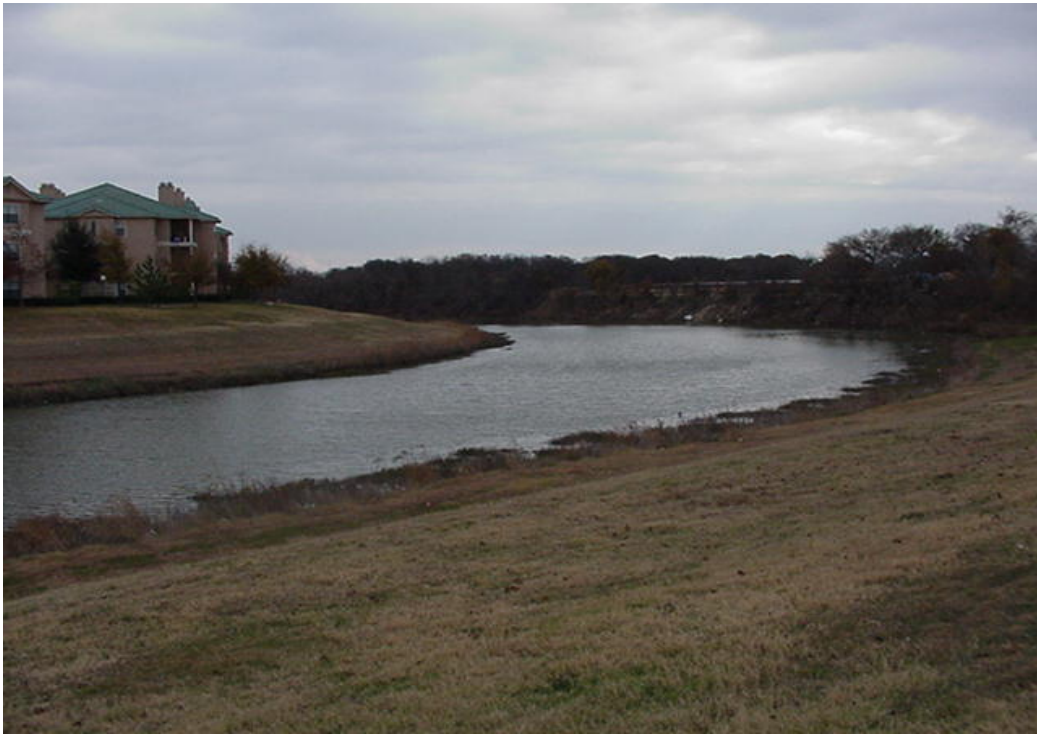
Figure 5. View of development along channelized bank of Big Fossil Creek.
