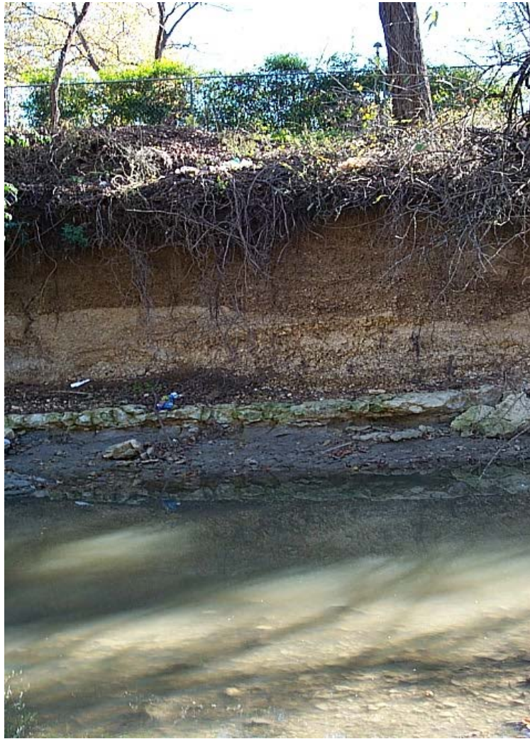
Figure 10. View of south cut bank, Little Fossil Creek.
