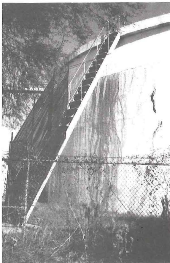
Figure 16. View north-northwest of the west side of the eastern Bedell tank, 1997.
