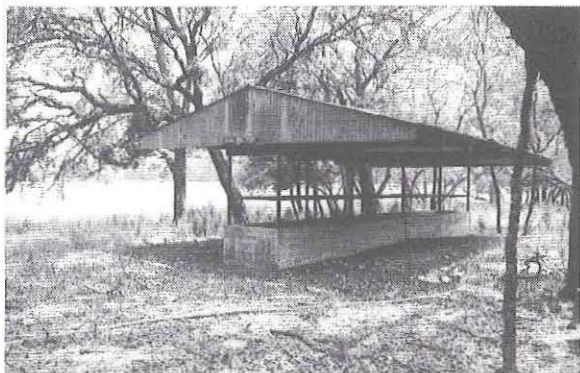
Figure 46. View to the northwest of Historic Resource No. 32d, feed trough.
