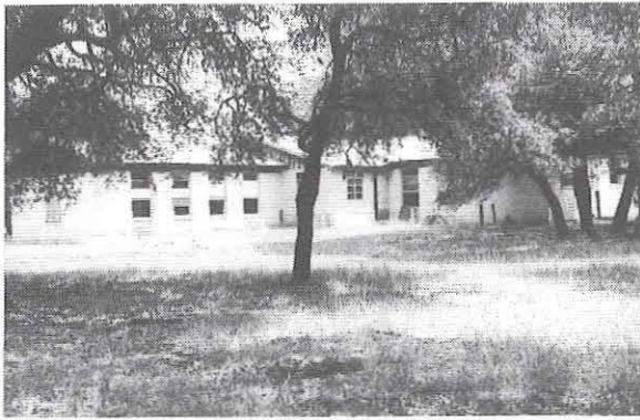
Figure 49. View to the southeast of Historic Resource No. 33, kitchen-dining room-dormitory.
