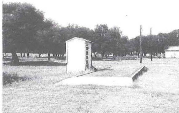
Figure 28. View to the southwest of Historic Resource No. 6b, truck scale.
