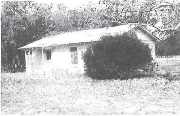
Figure 24. View to the northwest of Historic Resource No. 3, storekeeper/accountant's residence.
