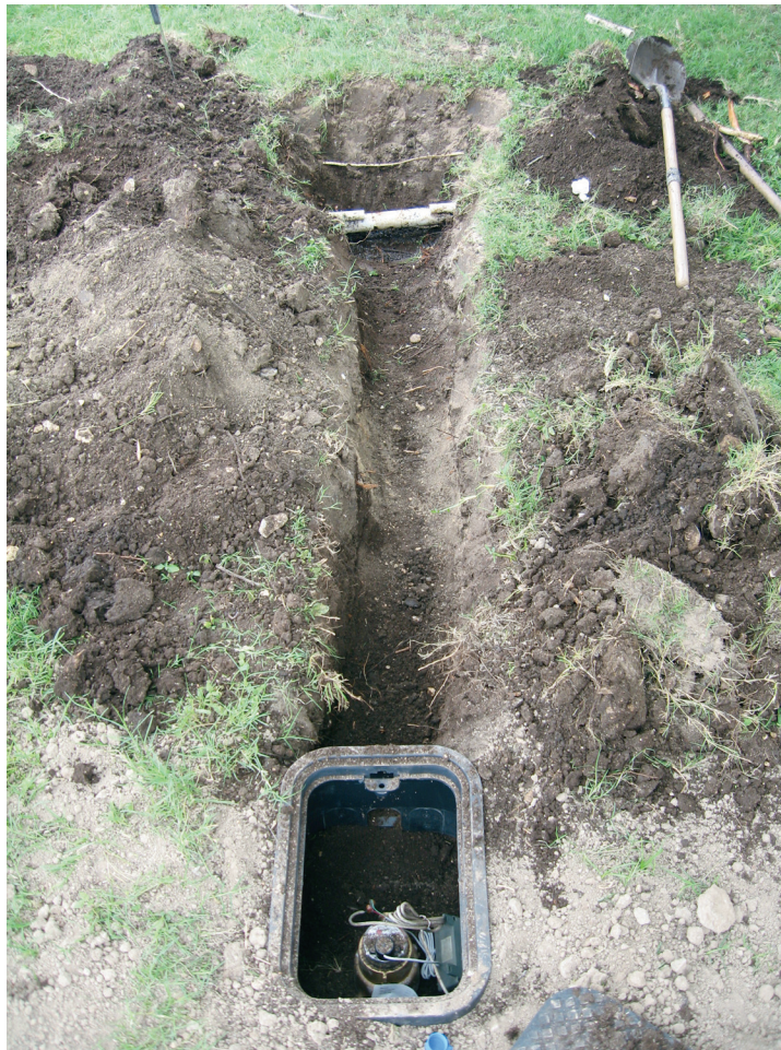
Figure 8-8. Meter box and trench, facing east.
