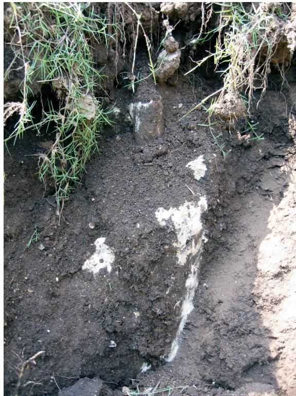
Figure 8-6. Closeup of a buried fence post with cement base.
