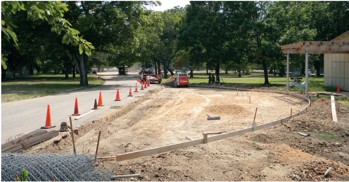
Figure 8-10. Overview of crescent-shaped access drive, looking southwest.
