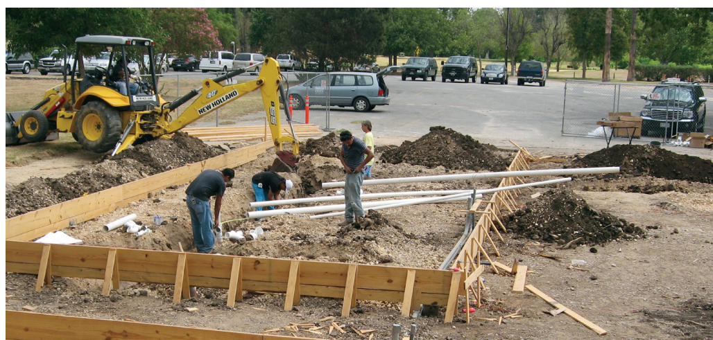
Figure 8-3. Overview of north building plumbing project, facing north.
