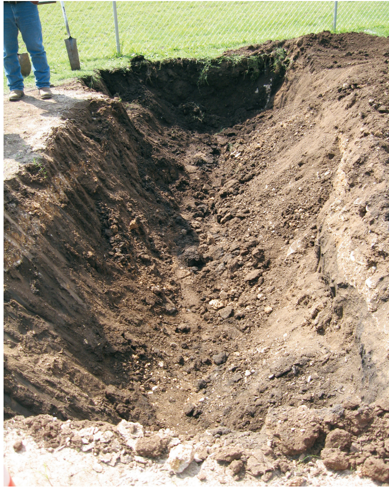
Figure 8-7. Exploratory trench for main water line, looking south.
