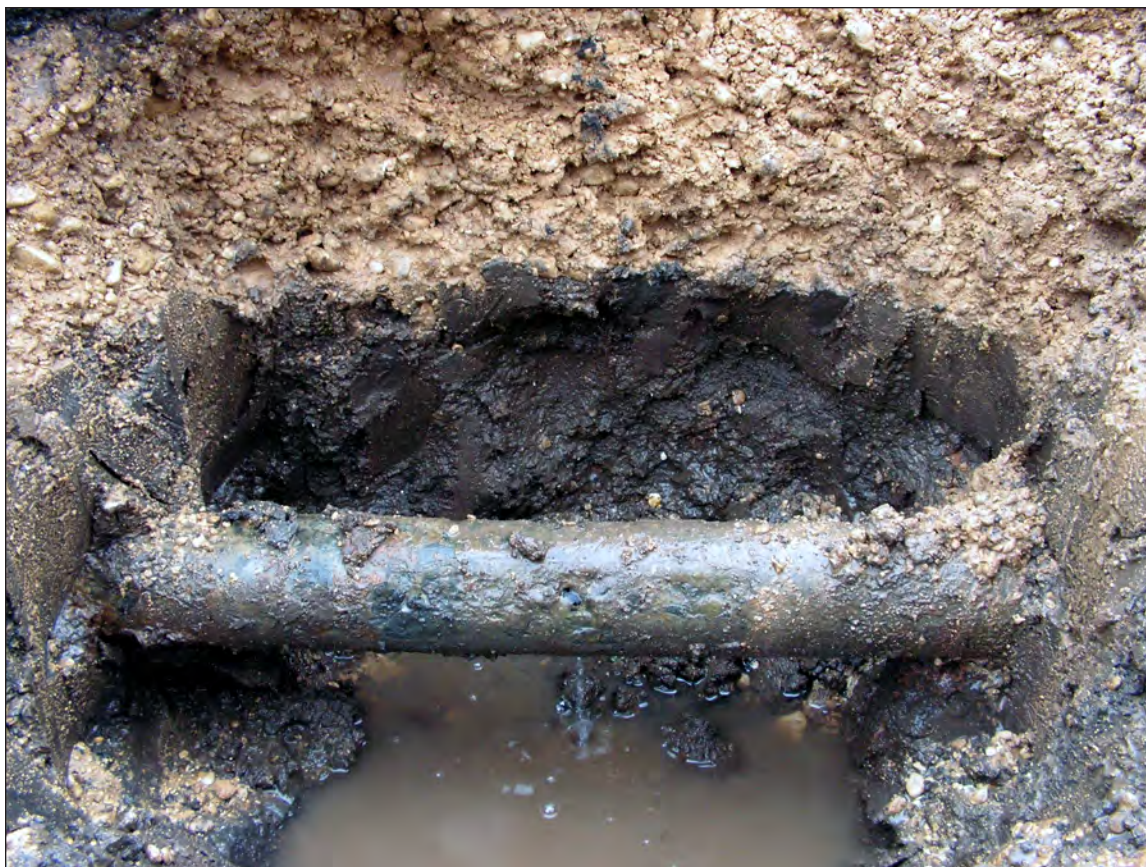
Figure 4-4. Exposed waterline.
