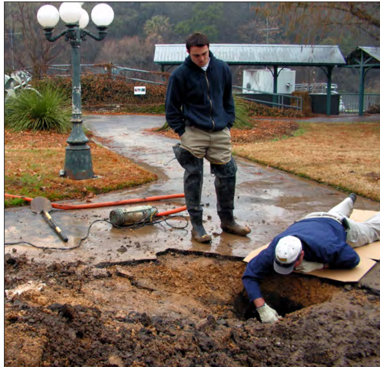
Figure 4-3. Continued excavation of waterline location.
