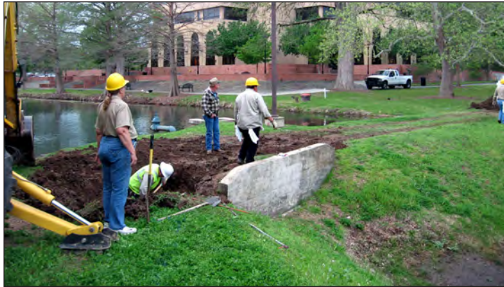
Figure 8-2. Texas State Facilities Services excavating Trench 2.
