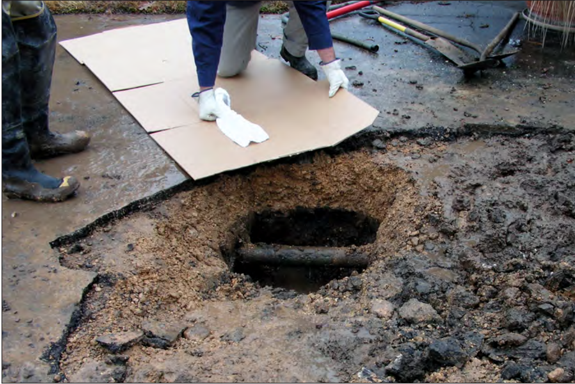
Figure 4-2. Excavation of waterline location.
