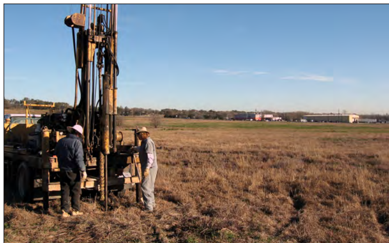
Figure 5-3. Geotechnical boring by Holt Engineering; facing north.
