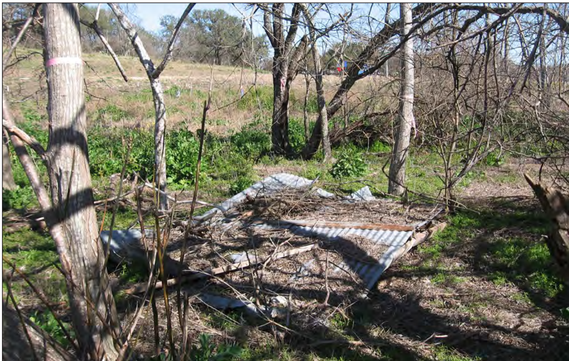
Figure 5-7. Collapsed metal-roofed shed.
