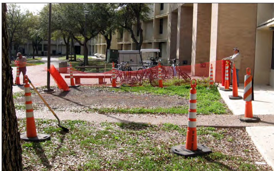
Figure 6-1. Trench location in front of Blanco Hall.
