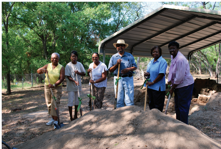
Figure 3-10. On August 4, 2008, Wilson Pottery Foundation members ceremonially threw the first shovels of dirt onto the beehive kiln to begin the conservation work.
