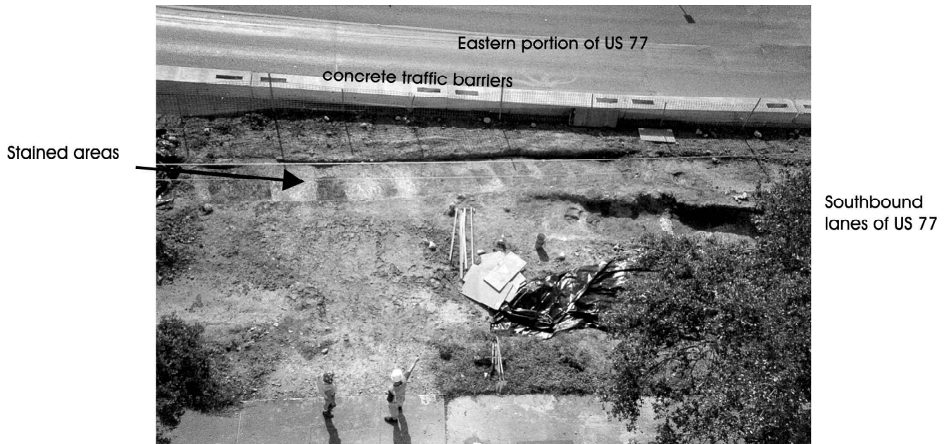
Figure 7-3. Area of burial investigations beneath southbound lanes of US 77. (Photograph taken from the bell tower of Our Lady of Refuge Church, looking east.)
