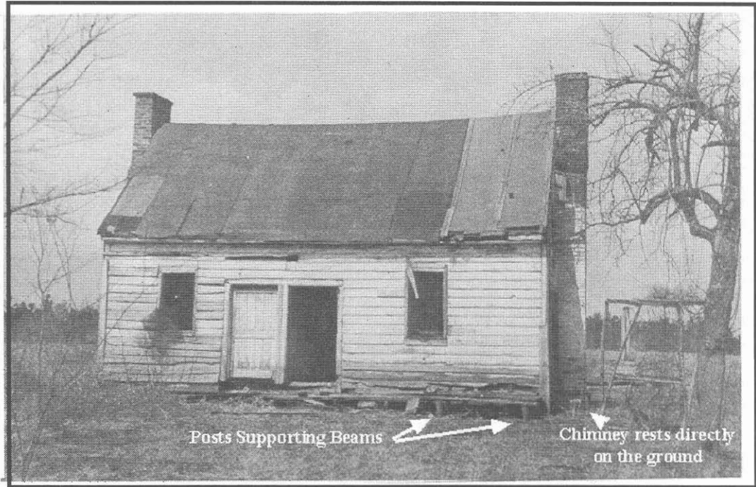
Figure 12: This is an example of post and beam construction with brick chimneys. The picture was taken by Thomas T. Waterman in 1940 and published in back of the Big House. The Architecture of Plantation Slavery by John Michael Vlach. This is a slave quarter from Henrico County, Virginia.
