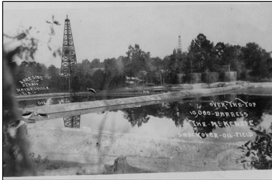
Figure 7. Historic photograph of lease pits near an oil well in the Smackover Oil Field (Culver & Barrett, 2001).
