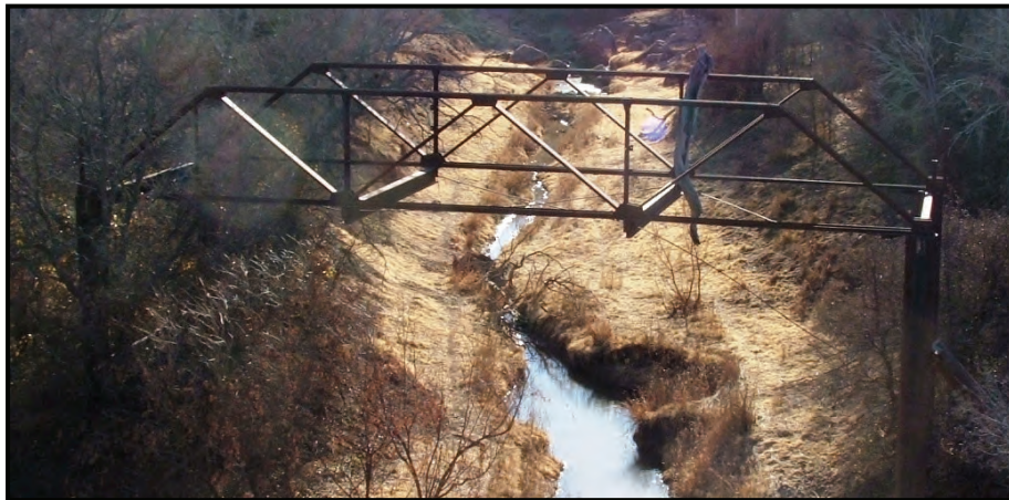
Figure 1-2. “Old Bridge 1” (41YN501) Crossing Gages Creek Adjacent to Site
