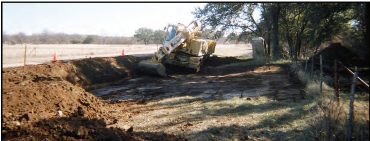
Figure 5-7. Gradall® Stripping South Block
