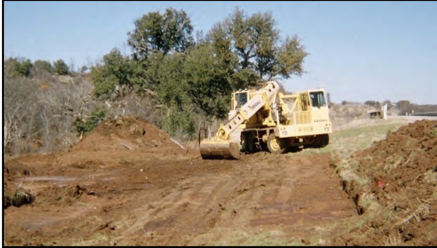
Figure 5-8. Gradall® Stripping North Block
