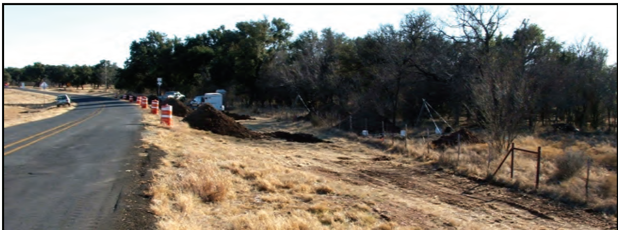
Figure 5-4. View of Trench Backdirt Piles Distributed along TxDOT ROW Containing 41YN452.
