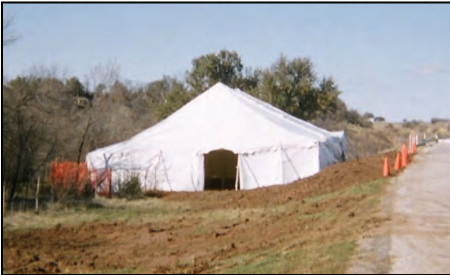
Figure 5-9. Tent Covering North Block
