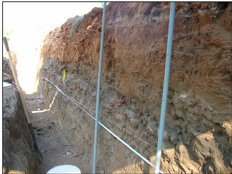
Figure 5.3. South elevation of BHT 1, opposite TUs 2 and 3. Note cultural material just above the string line (Feature 2); the yellow flagging tape indicates the location of a historic iron bar.
