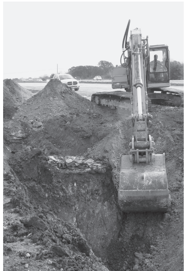
Figure 7. Well being isolated during excavation by trackhoe.
