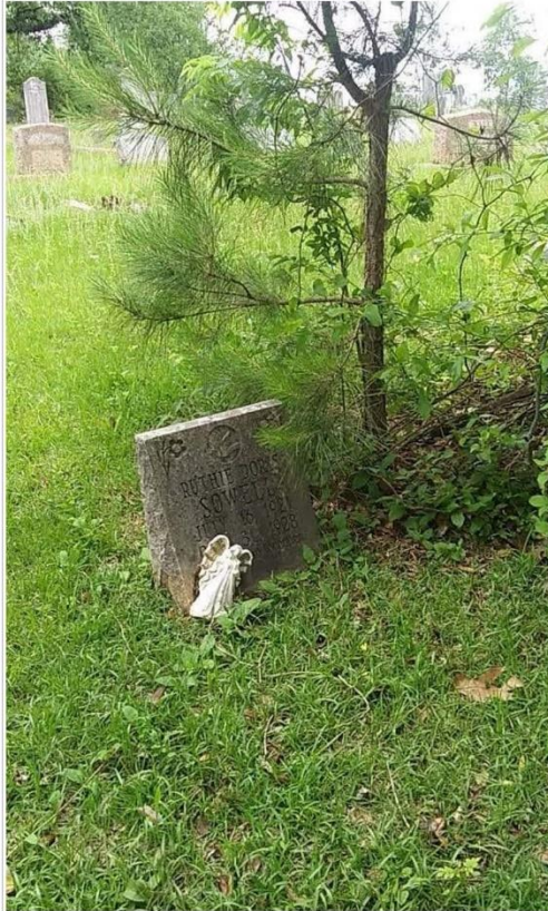
Figure 21: Though not necessarily intentional, this little pine tree is overtaking this gravemarker and gravegood because it has not been trimmed back properly or removed. This is at Attoyac Cemetery in San Augustine, Texas.
