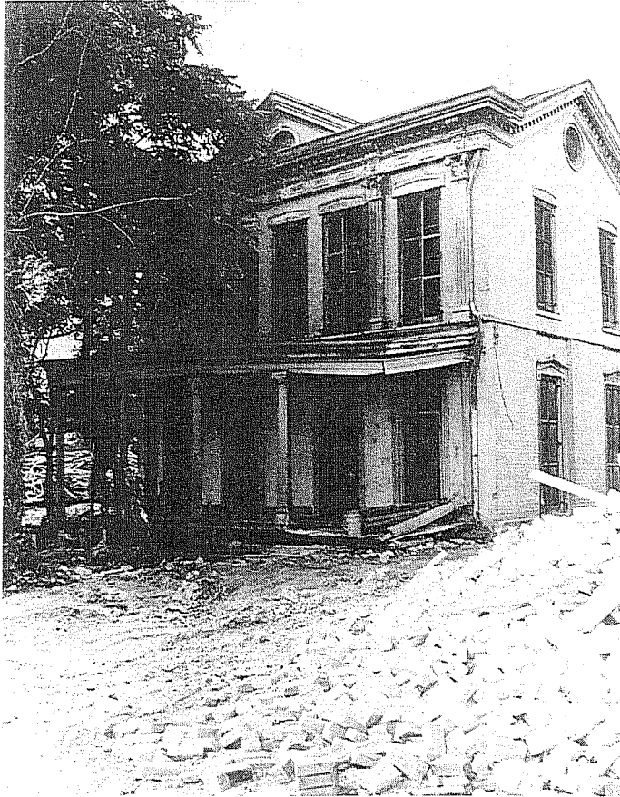
Figure A-21. Photo 20: Original Schultze House. 114 South Street. Demolished. (ITC Photo 82-587, ca. 1966)
