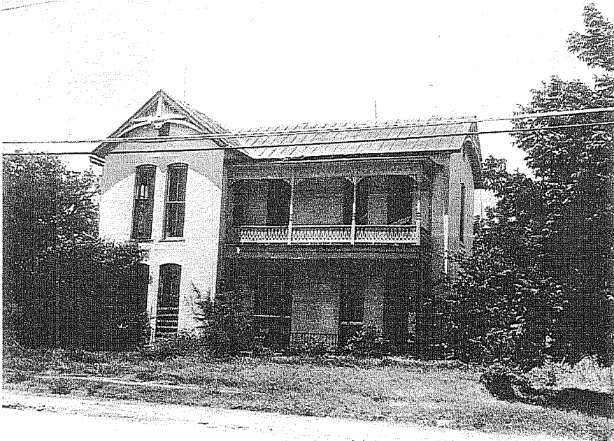
Figure A-12. Photo 11: 315 Goliad Street. Demolished. (ITC Photo 82-602, ca. 1966).
