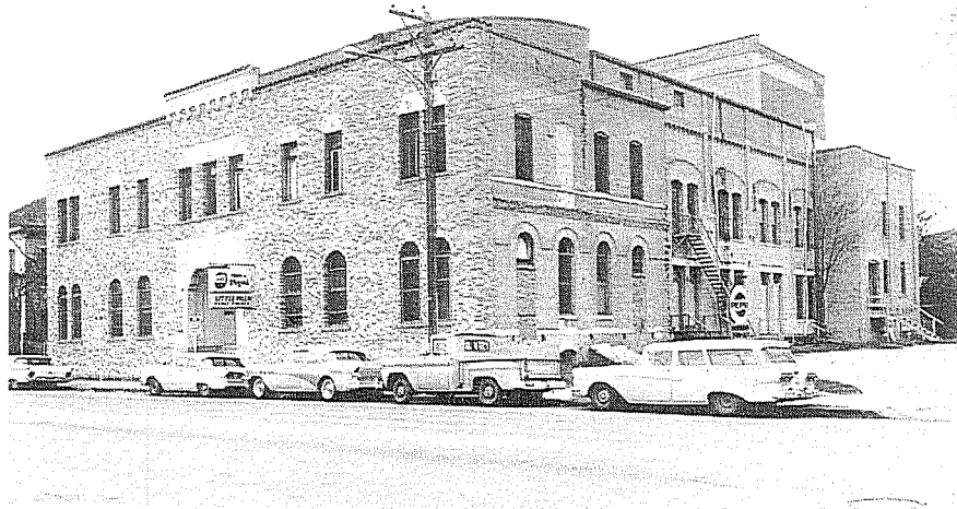
Figure A-2. Photo 2: Beethoven Hall. 418 South Alamo Street. Existing structure. (ITC Photo 82-574, ca. 1966).
