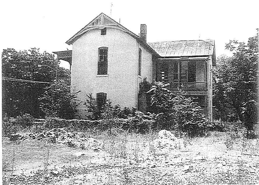
Figure A-13. Photo 12: 315 Goliad Street. Rear view. Demolished. (ITC Photo 82-603, ca. 1966).
