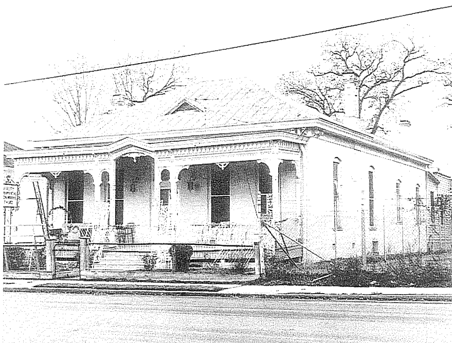
Figure A-23. Photo 22: Quality Ornamental Iron Works. 617 Water Street. Demolished. (ITC Photo 82-605, ca. 1966)
