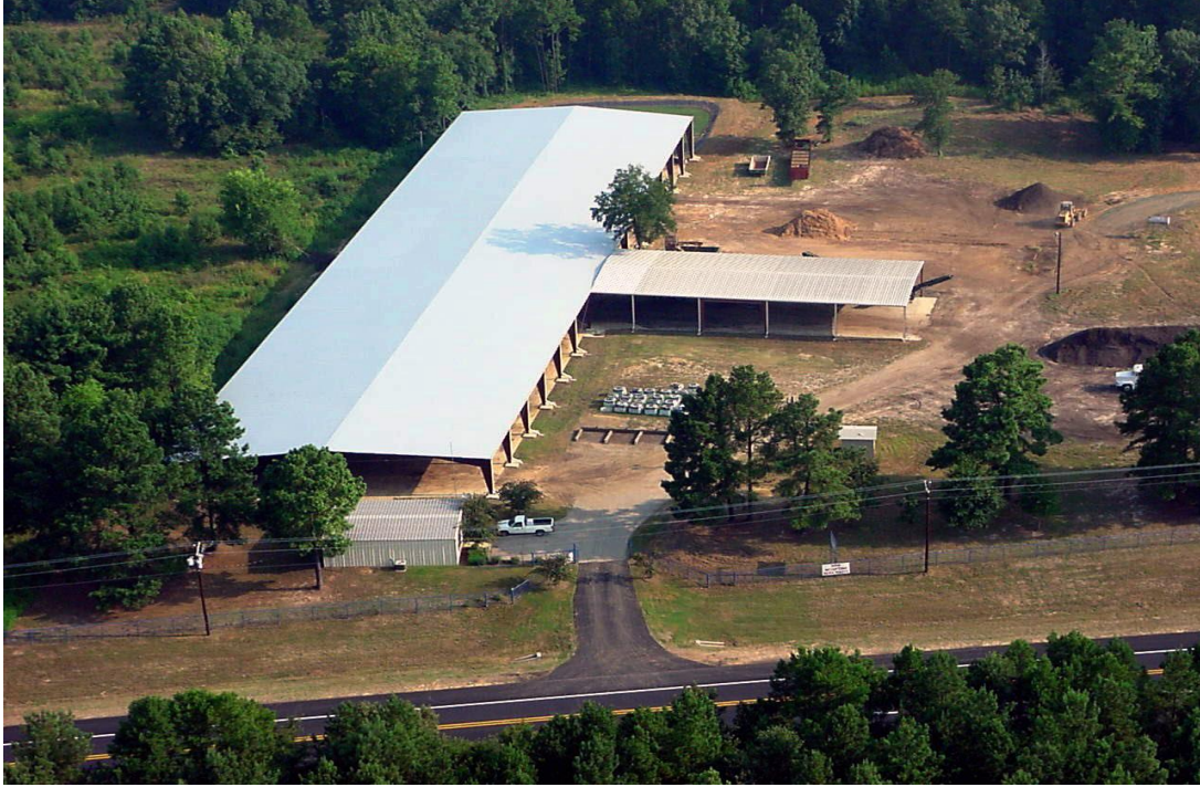
Figure 2.2: Aerial view of Angelina-Neches Compost Facility.
