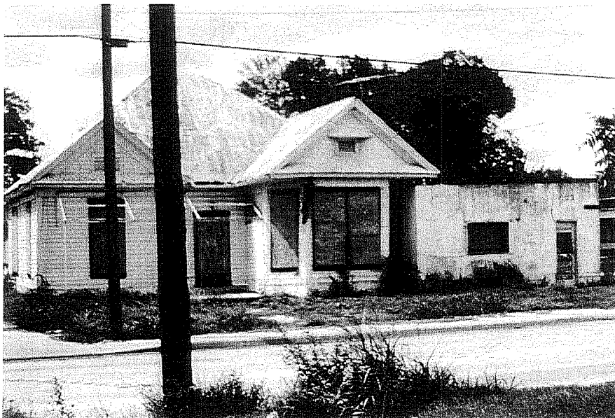
Figure 4-22. The Mendit Shop site.
