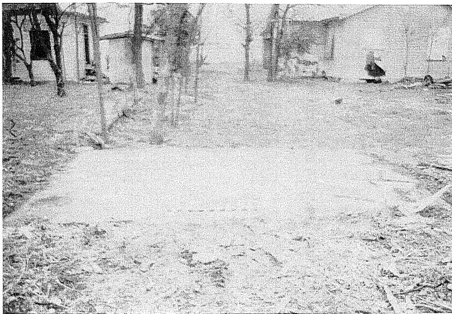
Figure 4-83. Excavation area for Trench D.
