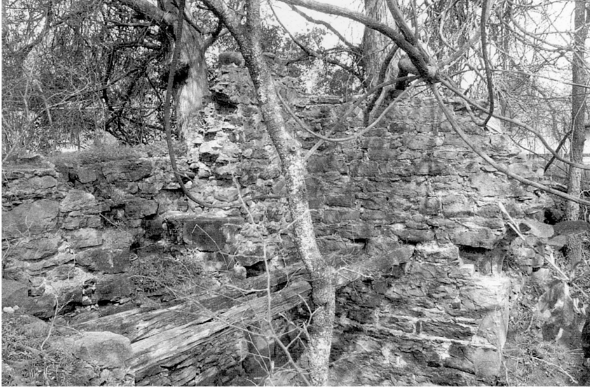
Figure 87. Aussilloux House showing remains of floor joists.
