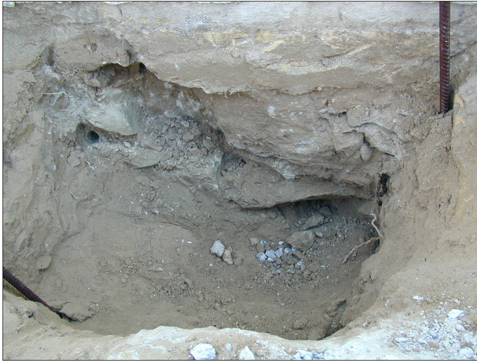
Figure 4-12. PSI Test Pit 7, outside the Ramirez Hospital, showing sandstone foundation.
