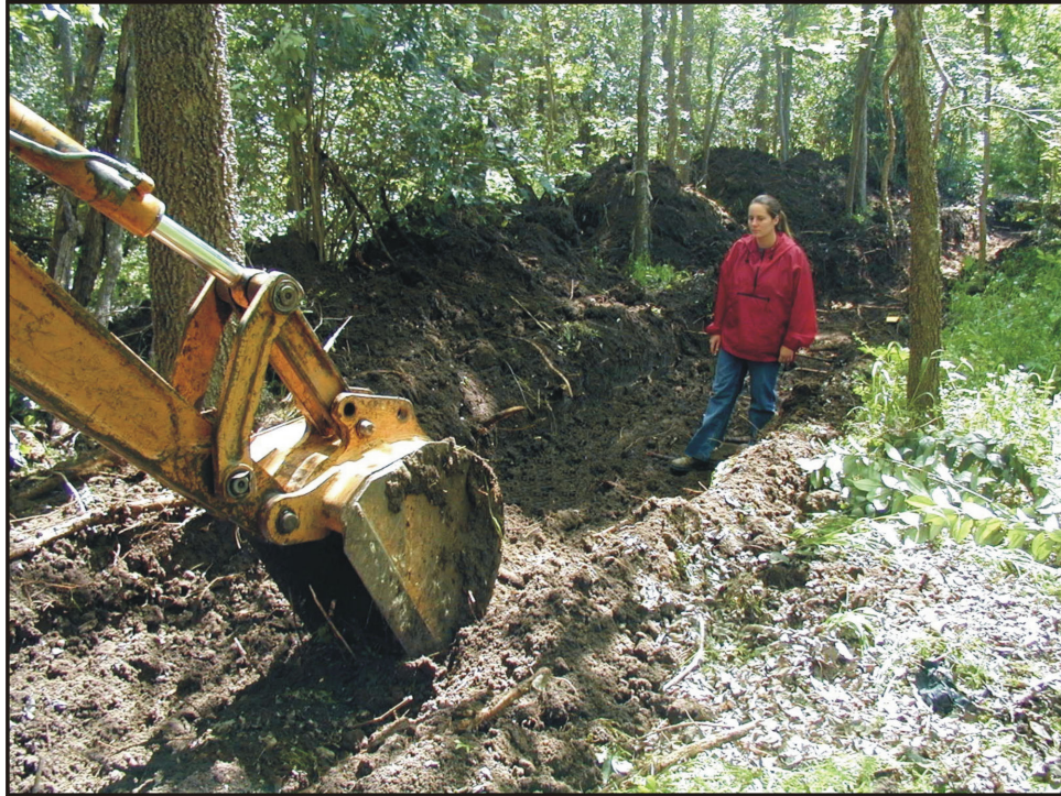
Figure 12. The excavation of Backhoe Trench 7.
