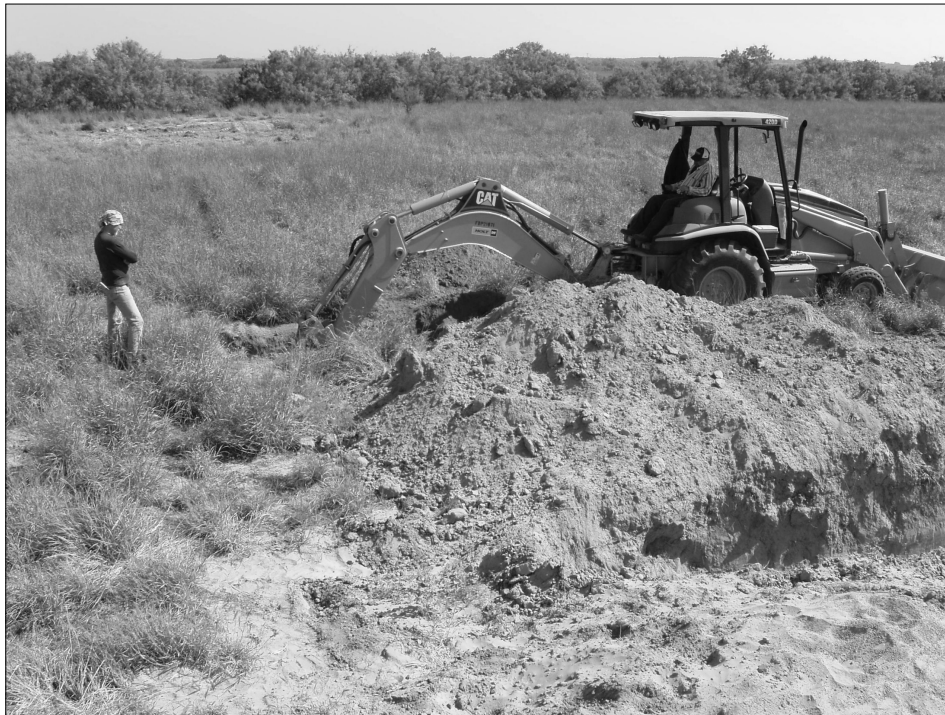
Figure 3-1. Backhoe trenching activities, Backhoe Trench 6-4 at Field Site 6.
