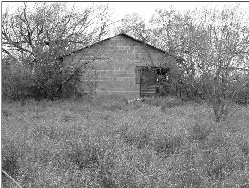
Figure 3-7. Brick structure located south of Field Site 3.
