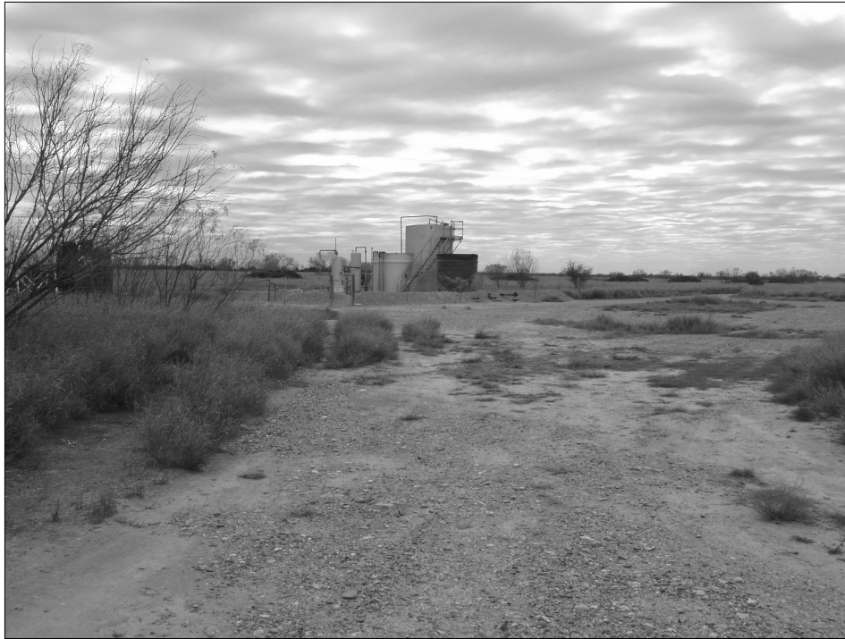
Figure 2-2. Operating well in the northwestern portion of the project area.
