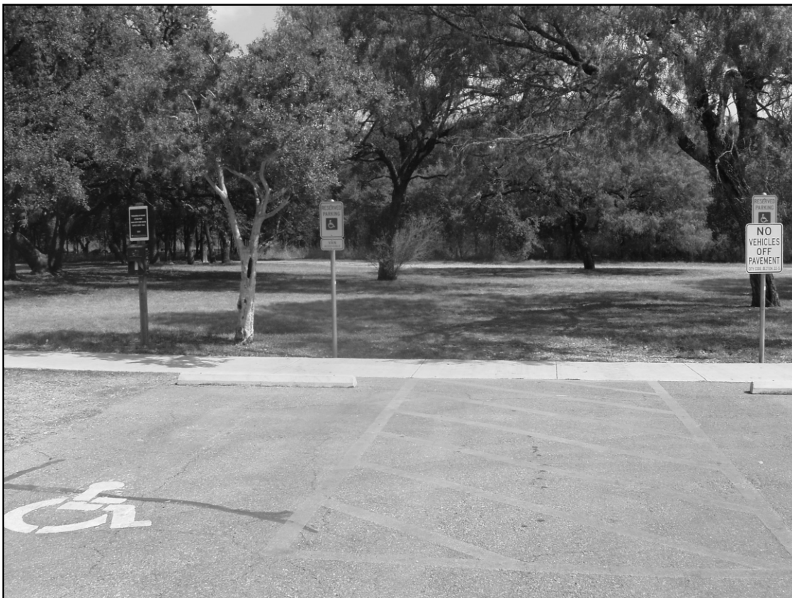
Figure 1-3. Parking lot and sidewalks in the vicinity of the new pavilion and playground in Area 1.
