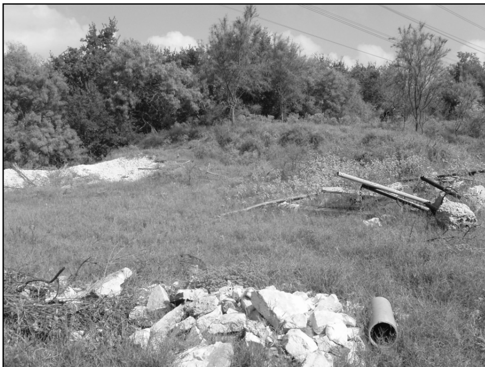
Figure 4-17. Construction debris and disturbance along the proposed water line in the northwest portion of Area 11.
