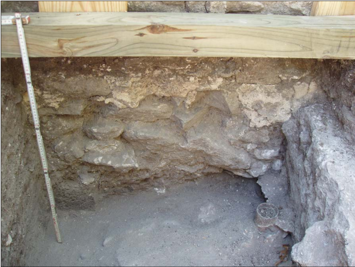
Figure 12. Photograph of the foundation.
