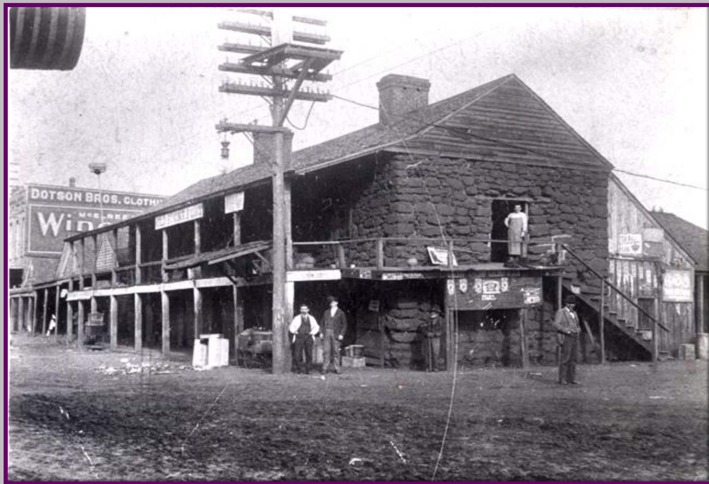
The first Nacogdoches County courthouse was the Old Stone Fort. This vernacular structure built in 1779 was also known as La Casa Piedra due to the Spanish rule over Texas which would continue for the next thirty years. It is easy to see the Spanish influence evident in the architecture of the Stone Fort; walls "made of brick similar to that used in the adobe houses of Spaniards".
