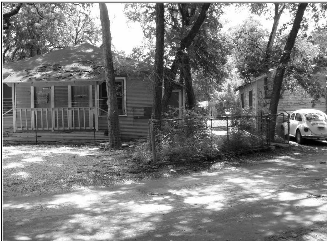
Figure 1-4. The San Antonio Parks and Recreation building.
