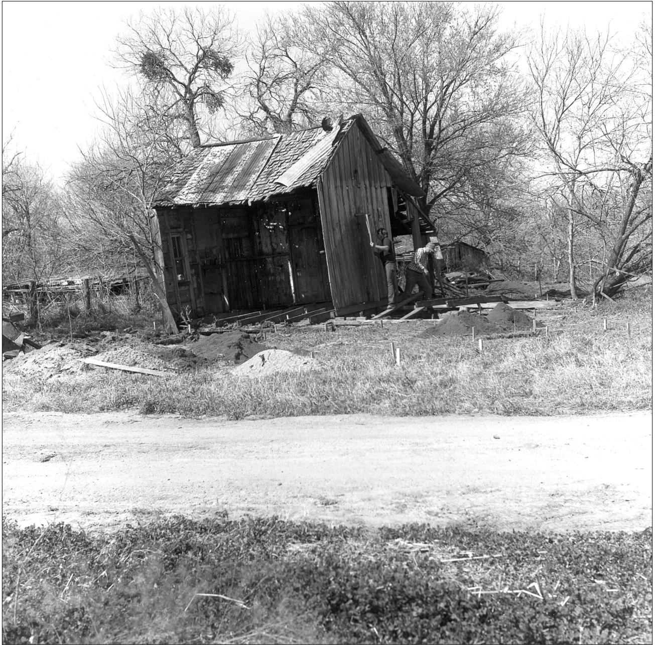
Figure 6. Photo of the Osborn tenant house taken February 1987.
