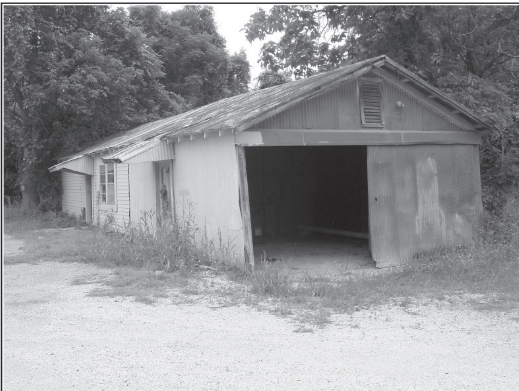
Figure 6-19. Second commercial structure at 1317 Farm Road.
