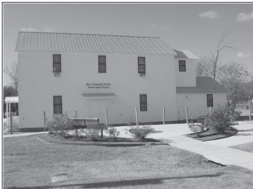
Figure 3-10. Kerr Community Center.
