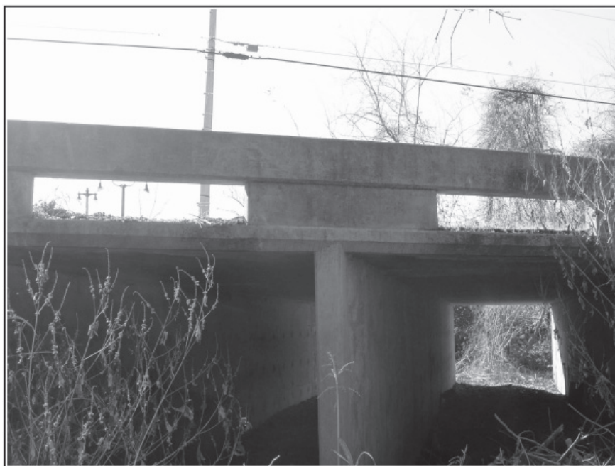
Figure 3-3. Current bridge over Gills Branch.
