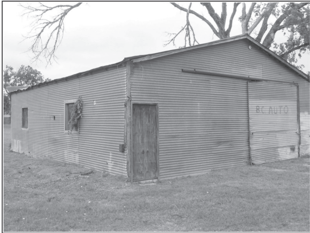
Figure 6-16. Commercial Structure at 910 Martin Luther King Drive.
