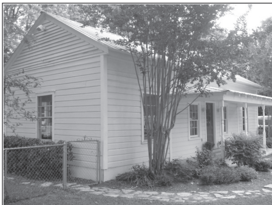
Figure 6-10. Historic residential structure at 1408 Chestnut Street.
