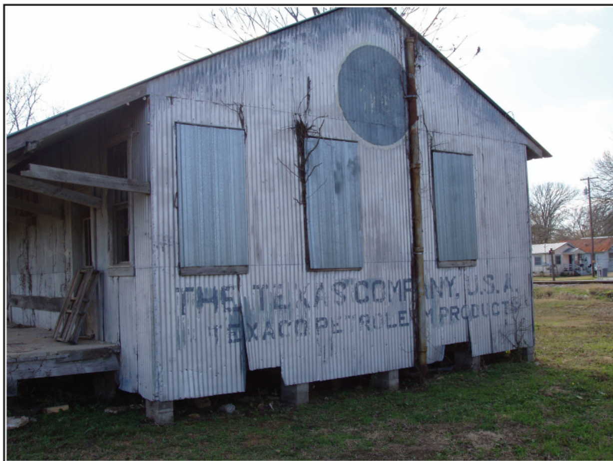
Figure 6-6. Company title adorning "The Texas Company" structure.
