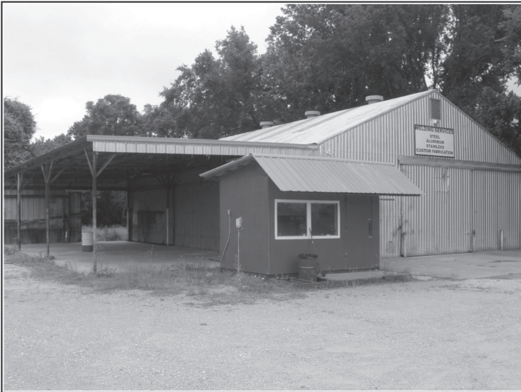
Figure 6-14. Commercial structures present at 1302 Chestnut Street.
