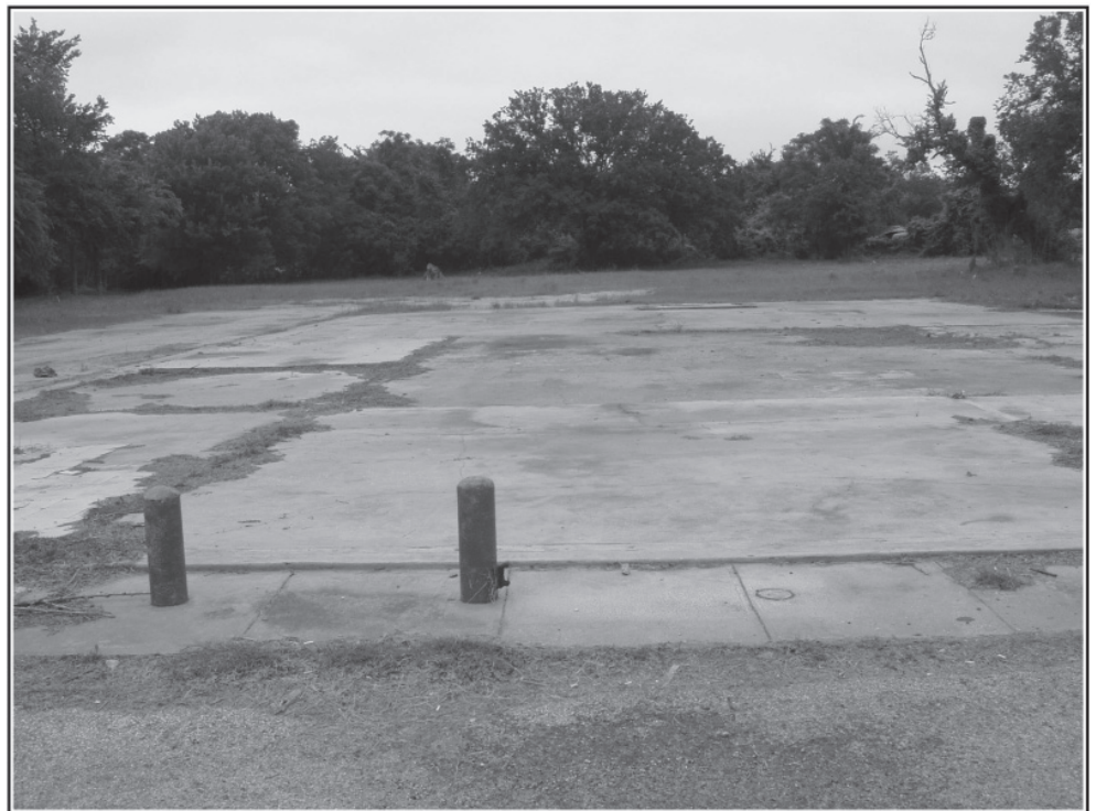
Figure 6-17. Foundation remnants of structure removed from 1404 Chestnut Street.
