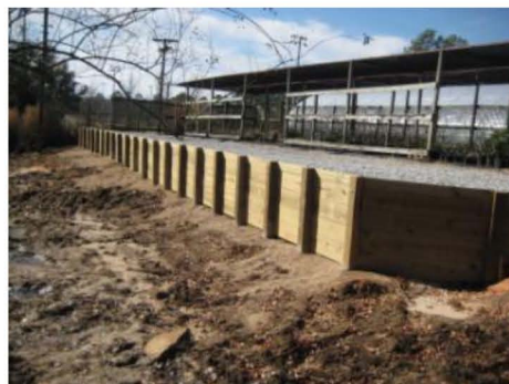
New retaining wall. What an improvement!
