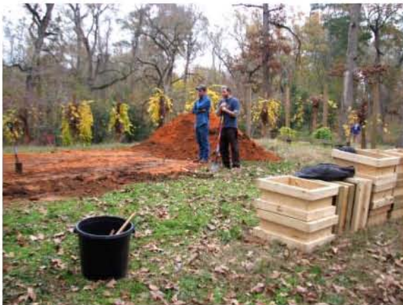
Jonathan Pickenpaugh and Trey Anderson survey the construction site of the future green roof pavilion at the PNPC
