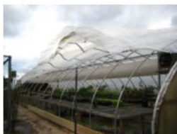
"Windows" in the poly house
