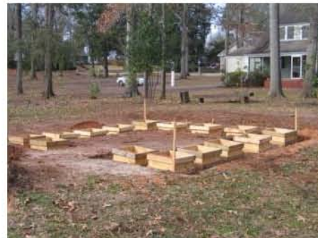
Forms for the support posts of the green roof pavilion
