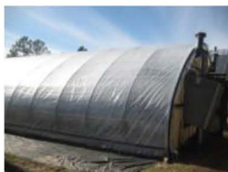
New greenhouse covering
