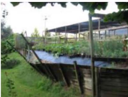
Old retaining wall
