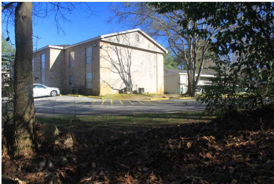
Figure 17: Image taken from Bonita Creek illustrating the lack of a levee and the relationship between Bonita Creek and the University Club Apartments. The apartments are 30 cm above the top of the stream channel. This allows flooding to occur on a regular basis.
