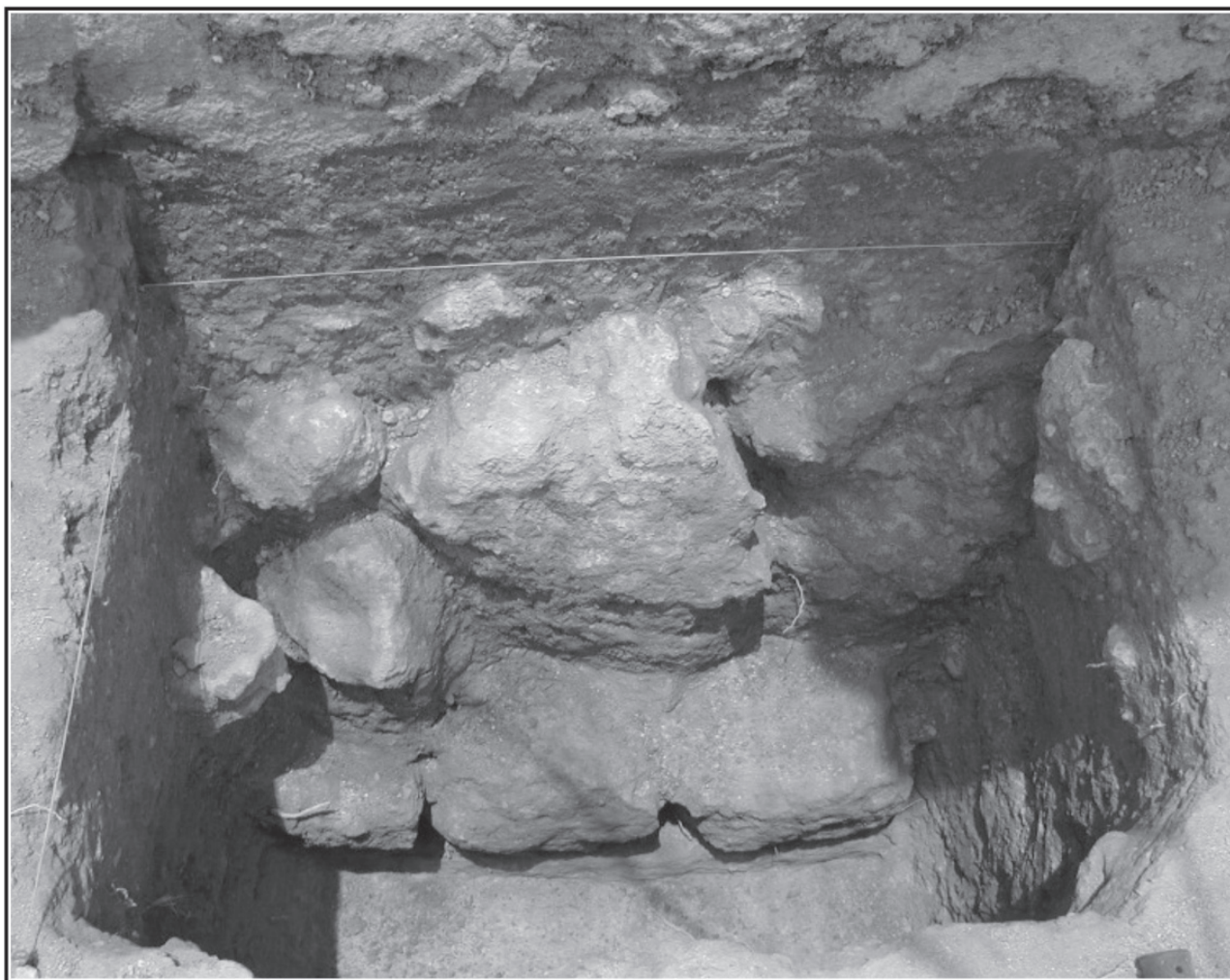
Figure 5-19. Foundation of Convento wall exposed in Test Unit 66.
