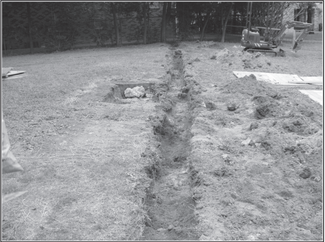
Figure 5-32. Southern portion of Trench 3 excavated by small trackhoe.
